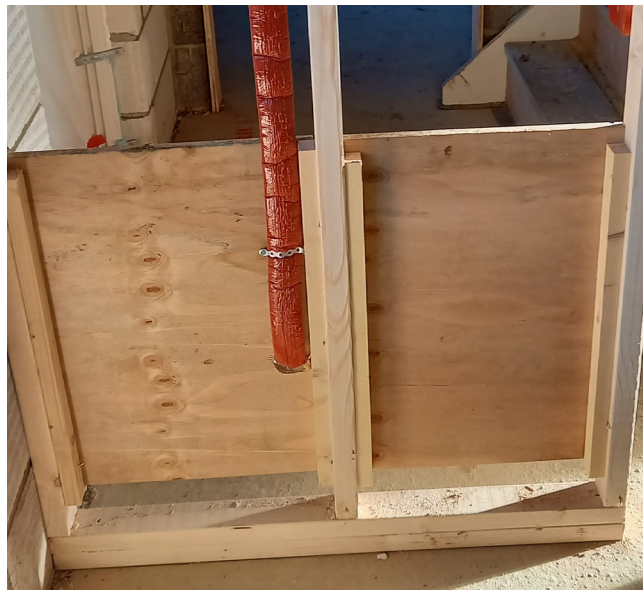
Attention to detail around this pattress work. Timber grounds have been correctly included to facilitate squarely driven fixings to ensure the element of support is well secured.
