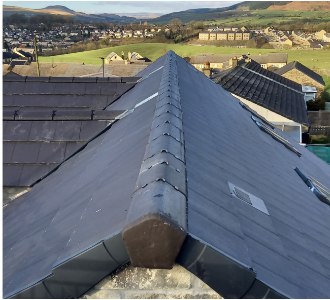
A dry ridge installation, all unions fixed and the use of a block end ridge tile alongside these proprietary verge units gives a good degree of security to prevailing winds on this exposed ridge line.
