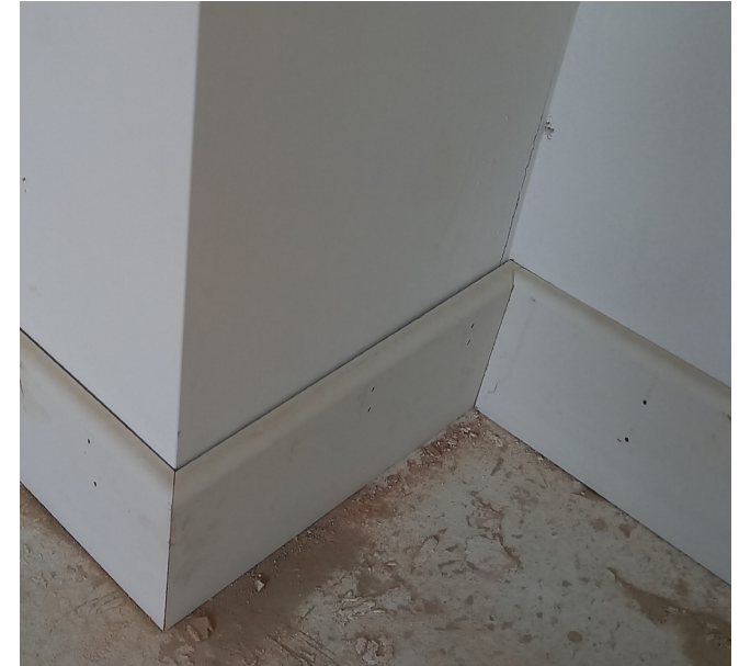
Skirting board with tight mitred external corners and internal corners accurately scribed to suit the section profile.
