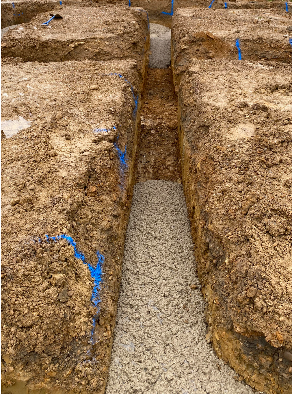
Concrete placement underway and being monitored against demarcation for fill levels.
