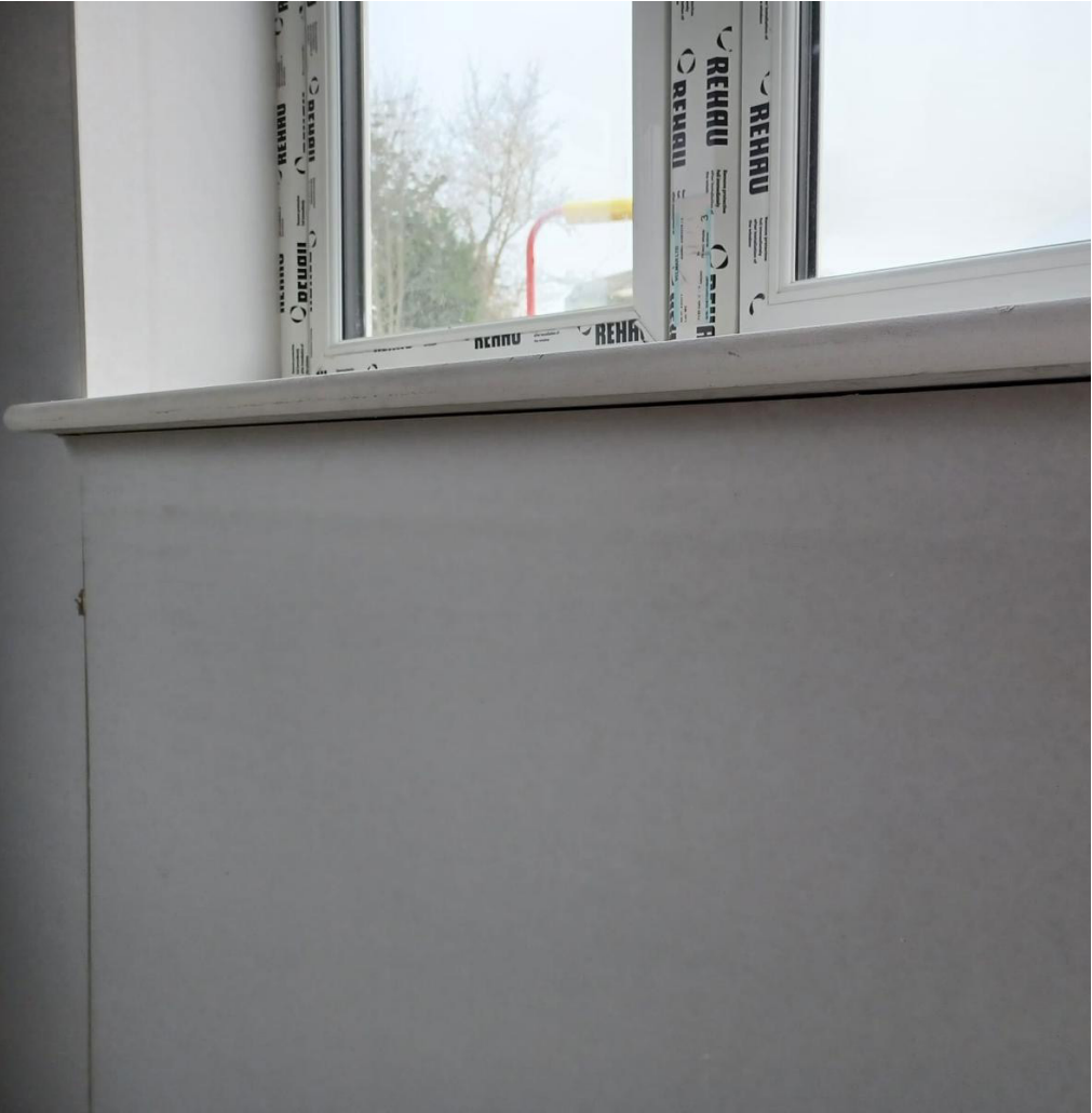
Well presented plaster board reveals with plumb and square board application, achieving equal margins to window jambs. Board termination under window board is neat and the gap is not excessive.
