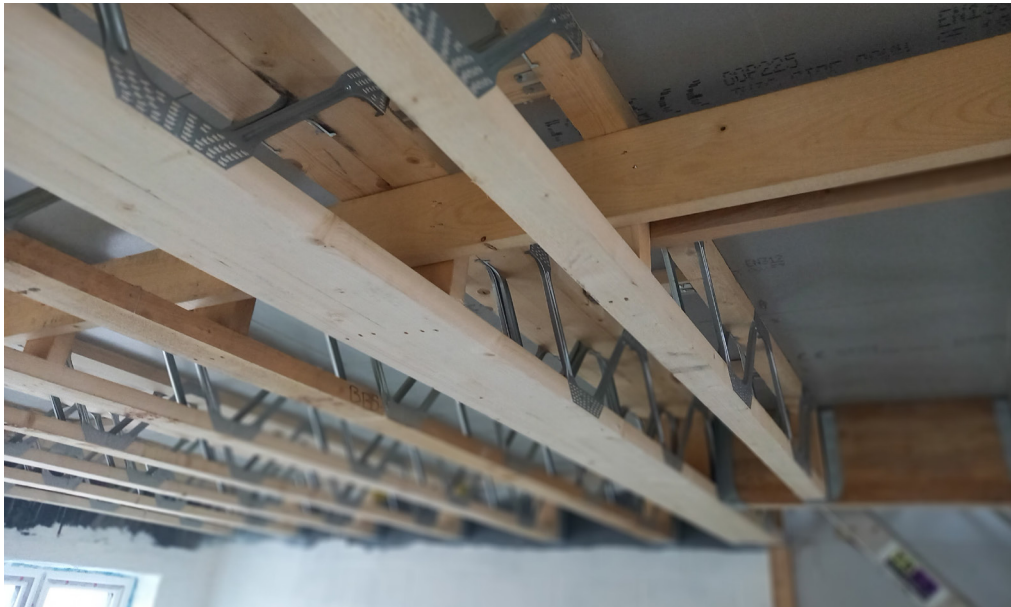
A timber strongback member in an engineered I-joist floor provides lateral stability and reduces deflection risk ensuring the floor system's overall strength and performance.
