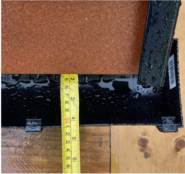
Eaves tile line has been correctly set to an overhang of 45mm when measured horizontally from the fascia. Importantly the proprietary preformed verge unit is aligned to discharge into the gutter ensuring no water collected in the verge unit misses the gutter.
