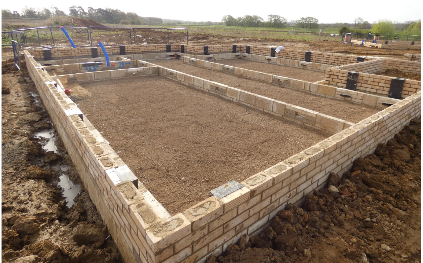
A cleared and well-presented plot ready for ground floor installation to commence.
