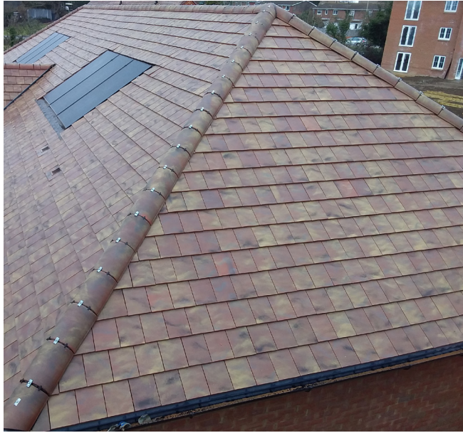
An example of a more complex roof covering installation – the appearance of the tile work is well blended. Hips and ridge work is installed to a high level and the often complex union is neat and well detailed to form good joints.
