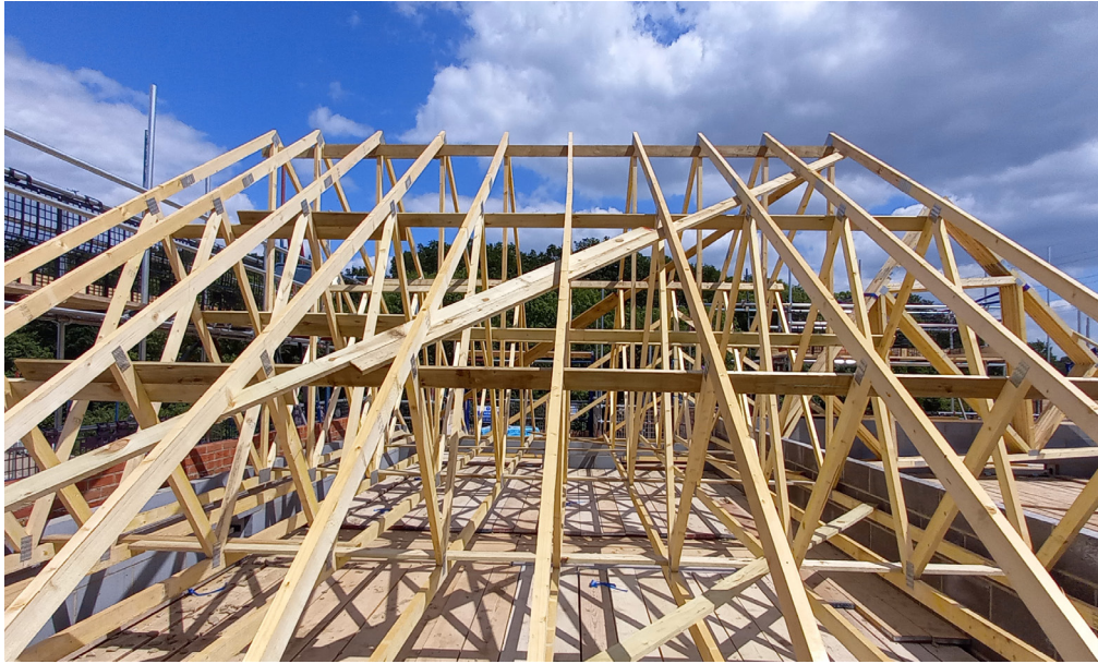
Trussed rafters being erected – longitudinal braces are fixed at the node points and diagonal bracing fixed into place. Unions in the bracing are correctly detailed with the side-by-side placement of bracing timbers to create continuity.
