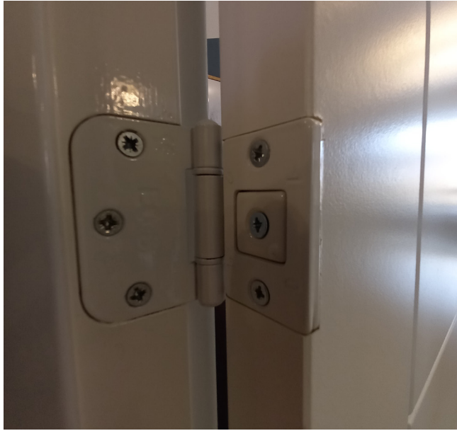
Great examples of well executed ironmongery installation – tightly fitted into accurate recesses, and free from scratches and damage.
