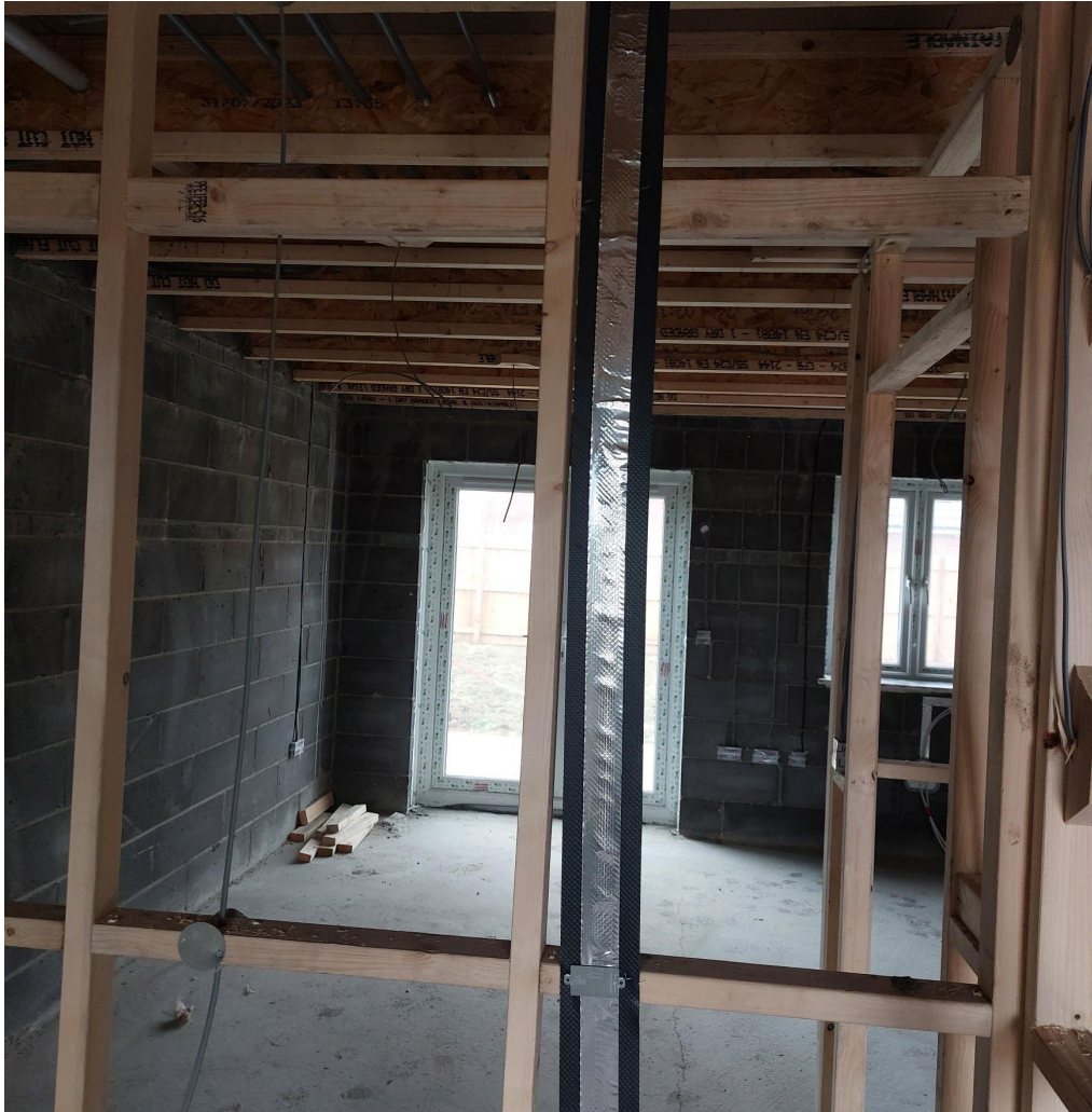
Metallic tracer tape applied to a DPC fixed over plastic pipe work to allow detection equipment to easily locate their position in service. The DPC avoids any issue created by tape adhesive and pipe material compatibility.
