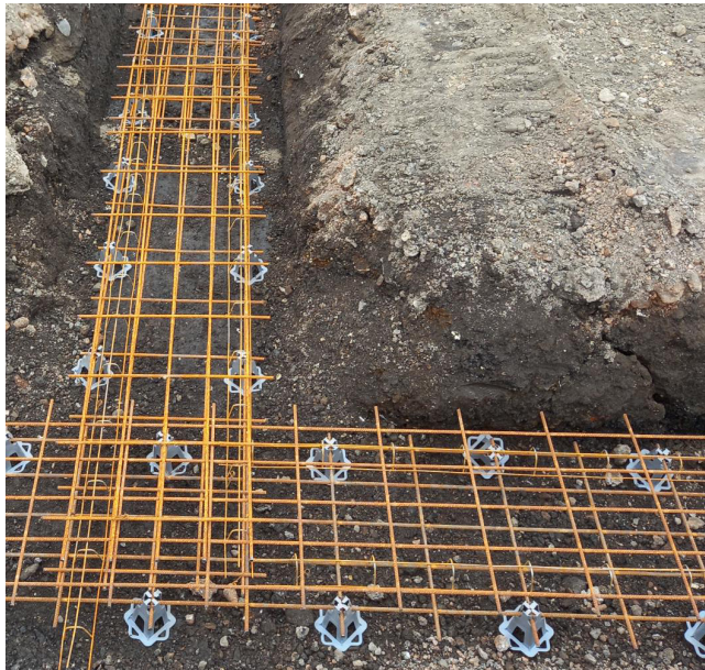
Correctly sized plastic supports to achieved a 75mm concrete cover as placed directly off strata. Wire stools holding apart layers to allow unobstructed concrete flow between the layers of reinforcement.
