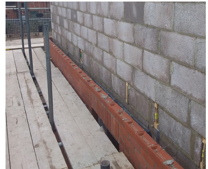
Concrete blockwork inner leaf with neatly struck off fully filled joints. A uniform pattern of wall ties can also be observed, coursed to allow follow on insulation boards to be placed.
