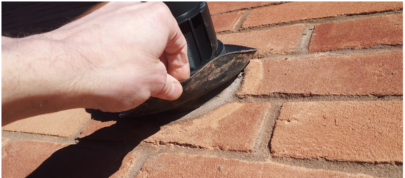
A boiler flue terminal with all gaps around the penetration pointed to create a seal prior to the proprietary flue collar being fitted.
