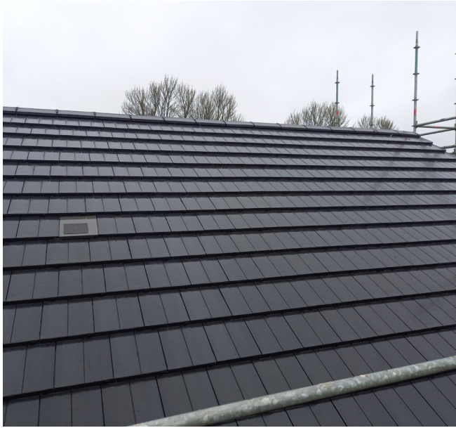
An example of a neat simple roof covering installation – tiles are installed to a good level and lateral shunt has been effectively utilised to ensure tiles are well gauged running into the verge to avoid small cuts. The ridge tiles are well aligned, fixed and levelled.
