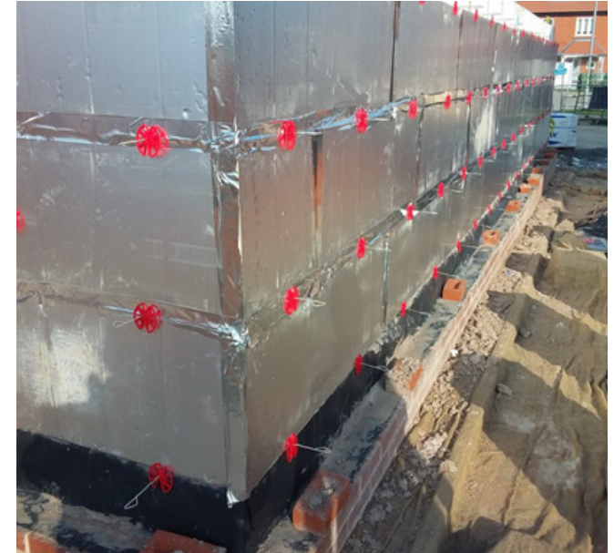
Rigid partial fill insulation boards, being installed with a high degree of detail and care. Proprietary retention discs secure the insulation in the cavity, and all board joints and ends have been foil-taped sealed.
