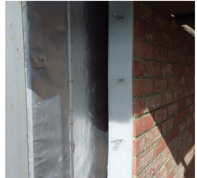
Proprietary slip ties built into the masonry panel at 225mm centres. Compressible polyurethane foam has been neatly placed, set back to facilitate follow on sealant to the correct depth.
