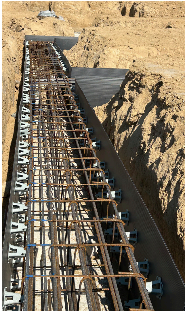
Ground beam work being carried out with consistent spacer positioning to facilitate the specified concrete cover.
