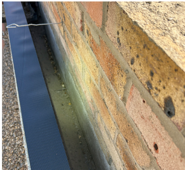
Maintaining a clear debris free cavity as work on the splash course progresses.
