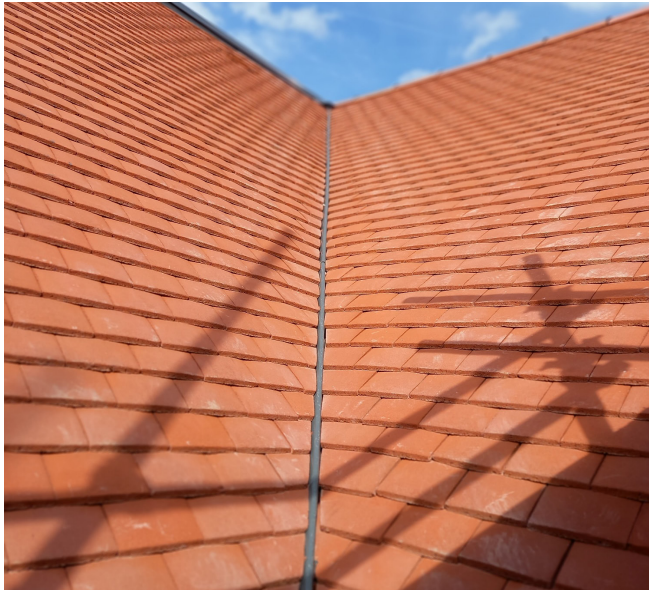
A neatly installed preformed valley. Tile lines are well aligned and cutting work neat and tidy.
