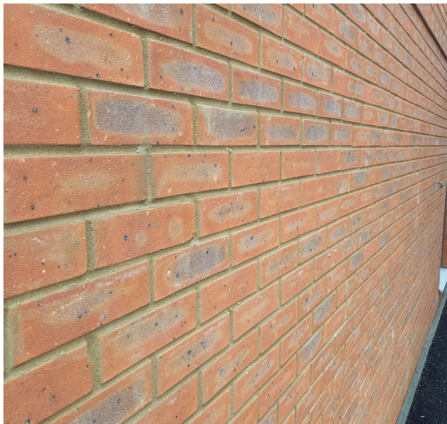
Neat masonry with joints that are well tooled and finished. Bed joints are uniform and level and perpendicular joints have a good vertical alignment.
