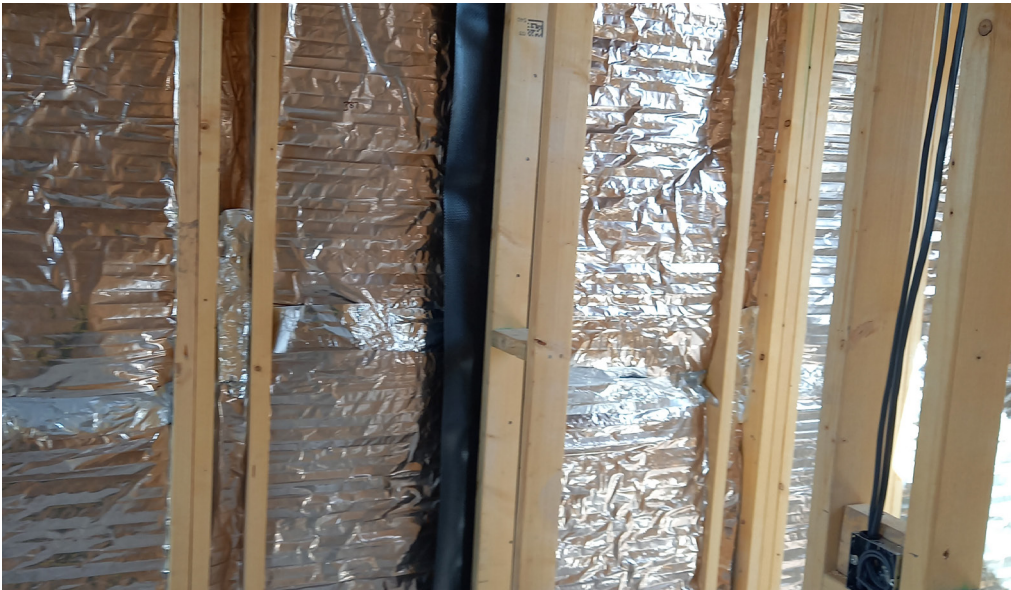
DPC material at the junction with the external wall and stud work to facilitate continuity of the AVCL within timber frame superstructure.
