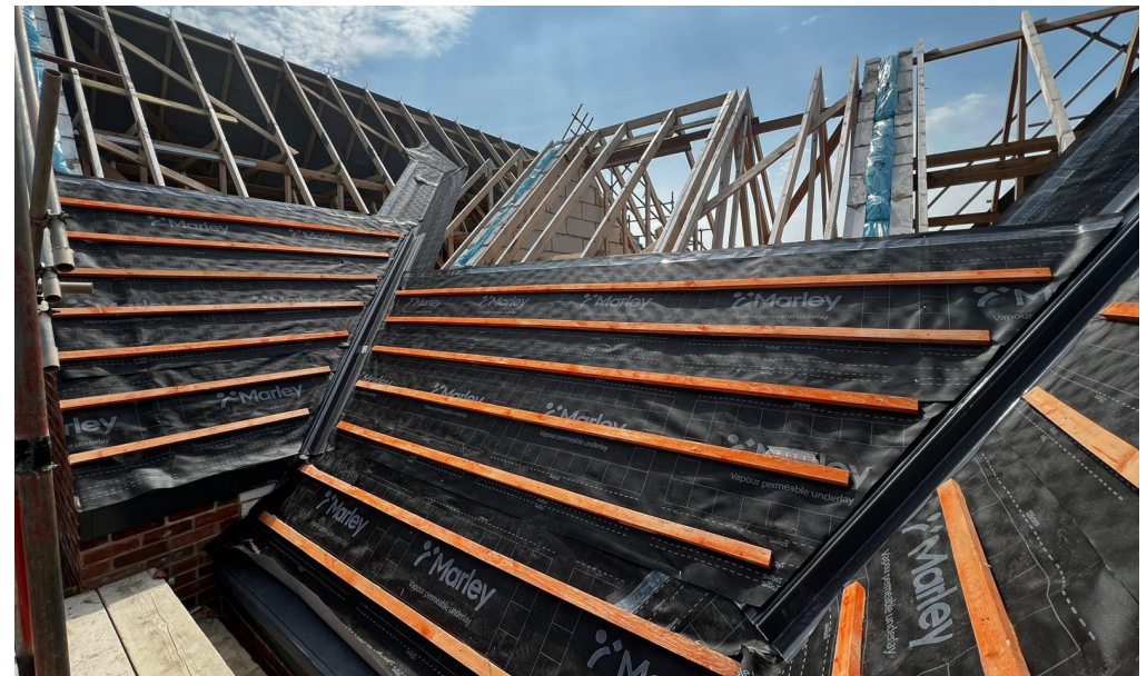
Proprietary valley linings being installed with underlay membrane dressed onto unit edges. The membrane laps are being taped sealed to negate the need for a battened lap.
