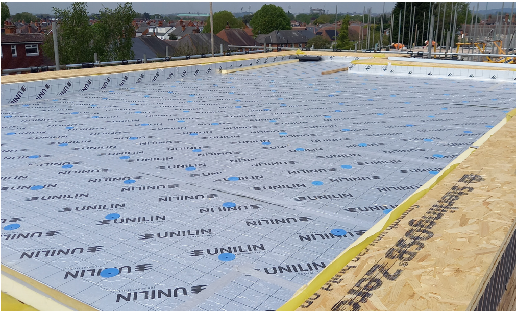
Ongoing work to a flat roof construction – rigid insulation installation in the warm roof configuration is well executed with staggered and tape sealed joints.
