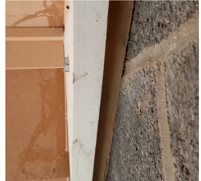
The wall string firmly secured to the adjacent wall with blocking included to ensure the string is in full contact with the adjacent wall when fixing.
