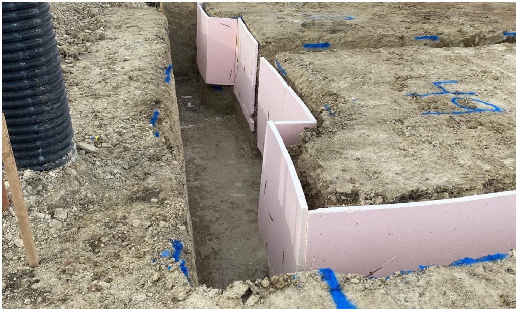
Heave precaution work being undertaken, fixed to the excavations vertical internal face in readiness for concrete placement.
