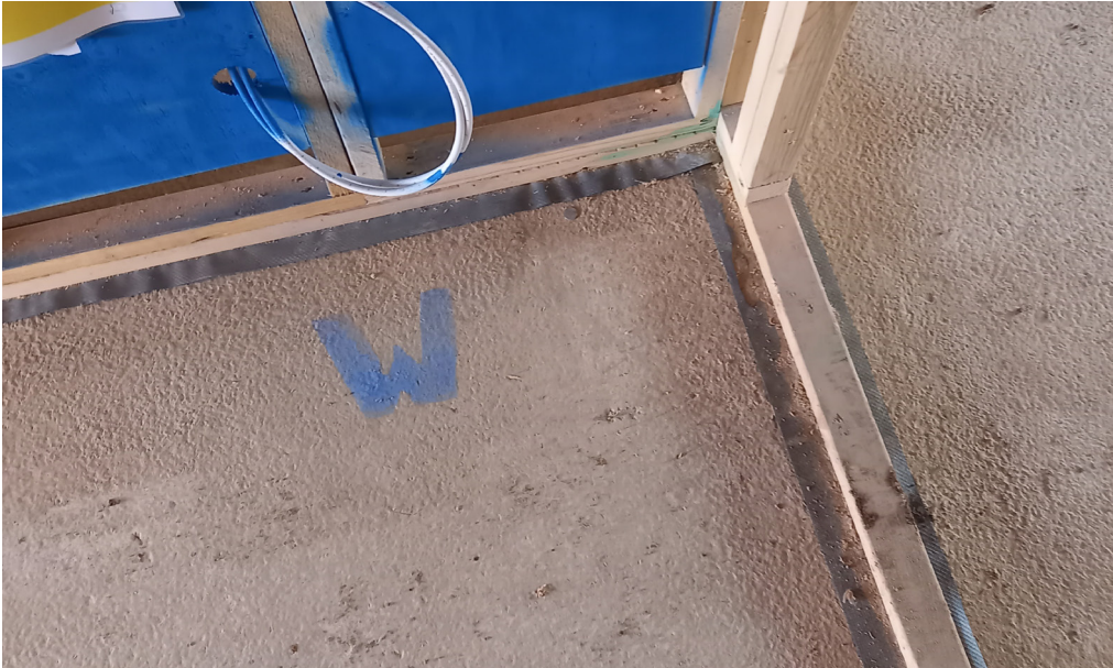
DPC material installed beneath the bottom rail of the stud work to safeguard against construction moisture transfer from screeds.
