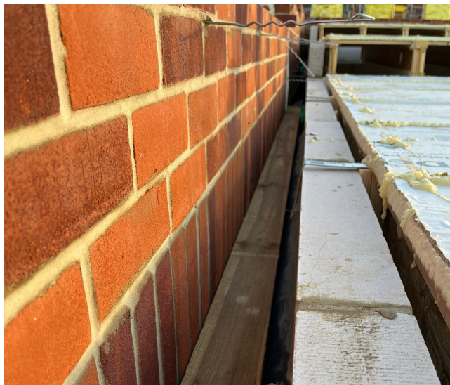
External leaf cavity face has been cleanly struck with filled joints. A cavity lath has been used to catch mortar debris as the inner leaf is built. Proprietary metal strap restraints at the junction with the intermediate floor are being accurately built into inner leaf at maximum 2m centres with a section of the strap returning tightly down the cavity to provide points of restraint.
