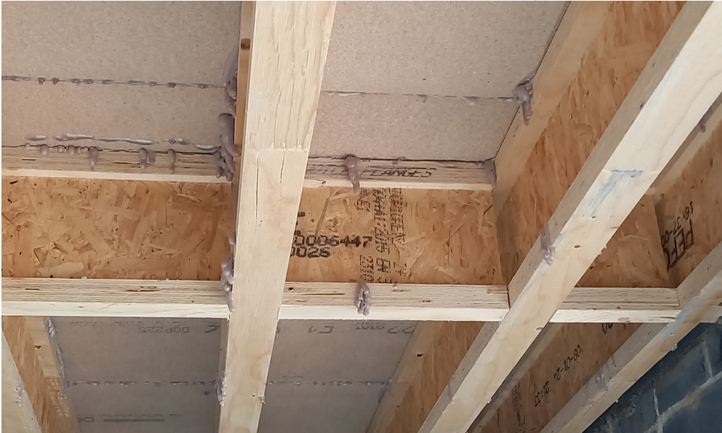
Full depth nogging work completed on this engineered I-joist floor. The lateral restraint is set on top of this nogging arrangement to restrain the parallel masonry as required.
