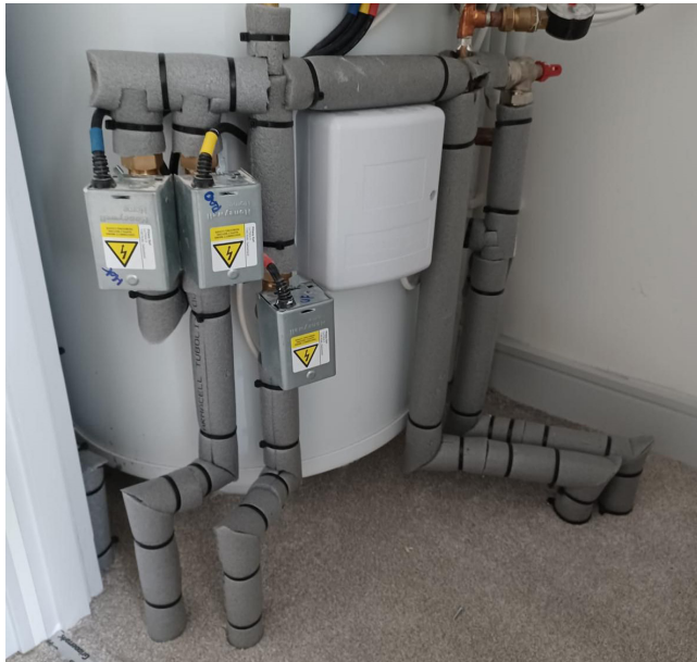
Exposed pipe work in these heating appliance cupboards has been fully insulated. Insulation material secured with cable ties and all joints neatly formed.
