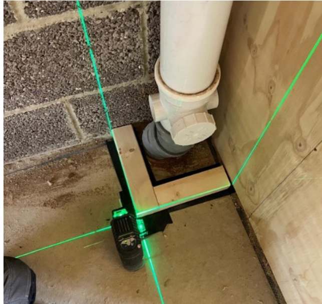
Attention to detail in the setting out process to ensure the boxing into the SVP in square and plumb when fixed.
