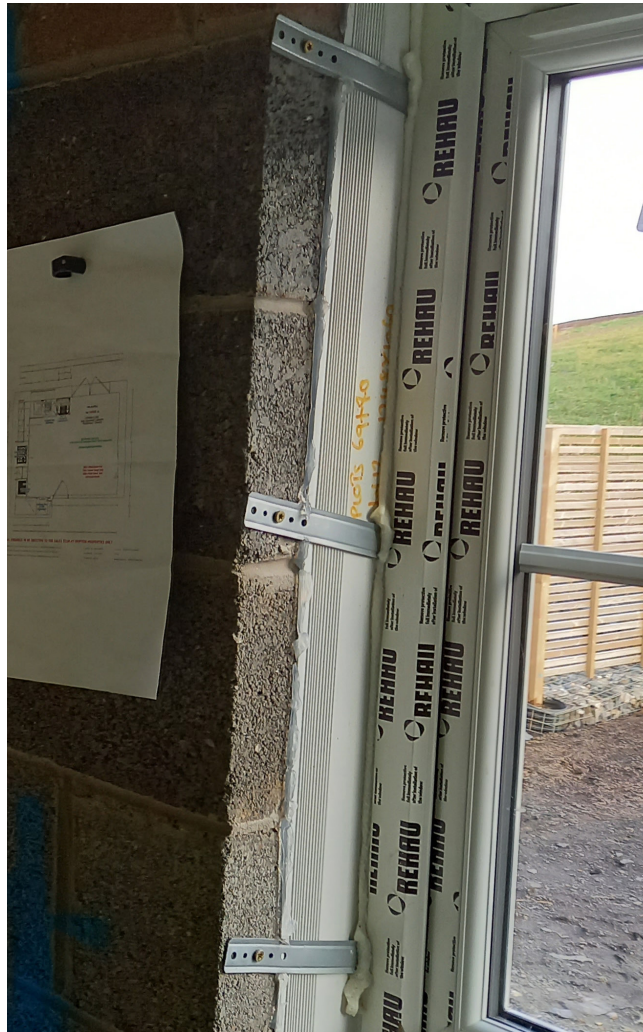
Proprietary fixing brackets installed to secure frame to appropriate surrounding masonry reveal without distortion to the frame.
