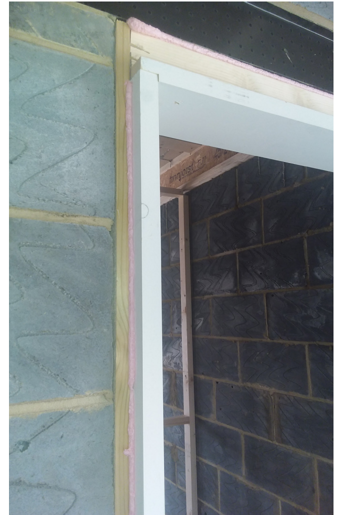
A door casing with solid timber continuous packing used to close fitting gaps to the structural opening. An expanding filling foam has been used to offer additional fixity in between mechanically fixed points.
