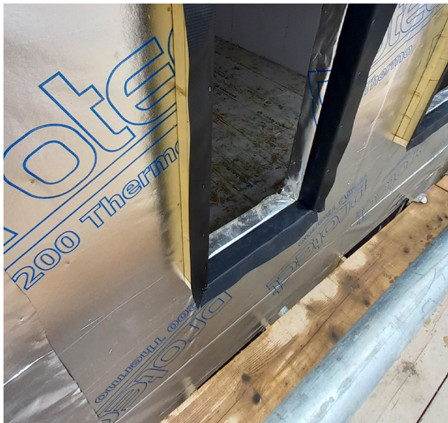
Timber cavity barriers have been installed to close off the cavity around openings. The treated timber section has been fully protected by a DPC, fixed and neatly detailed at corners and junctions with the breathable membrane in the opening reveal.
