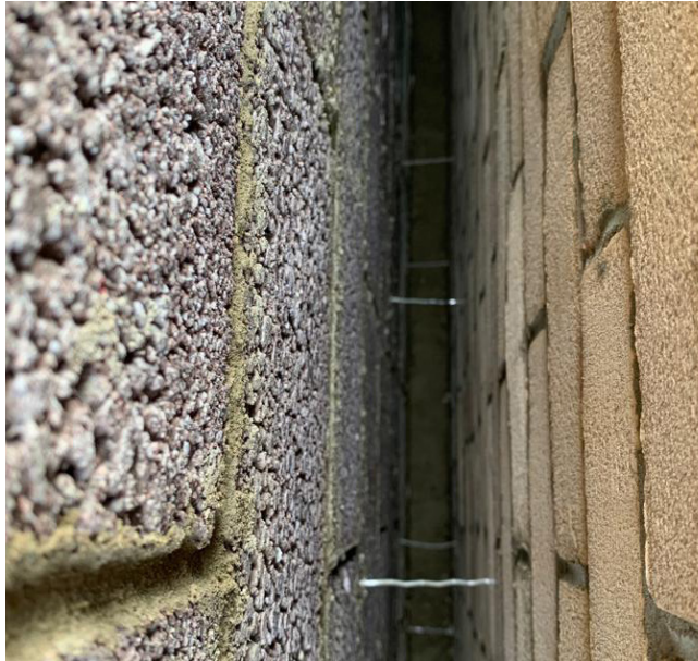
A view into the cavity of this well constructed masonry wall shows a clean cavity. Wall ties are also clean and all joints are filled and neatly tooled.
