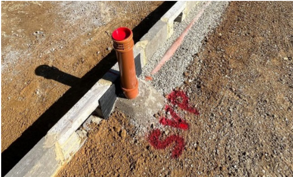
Concrete bedding being used to secure and hold rest bends to avoid accidental displacement during ground floor work with drains exhibiting good lines and falls.
