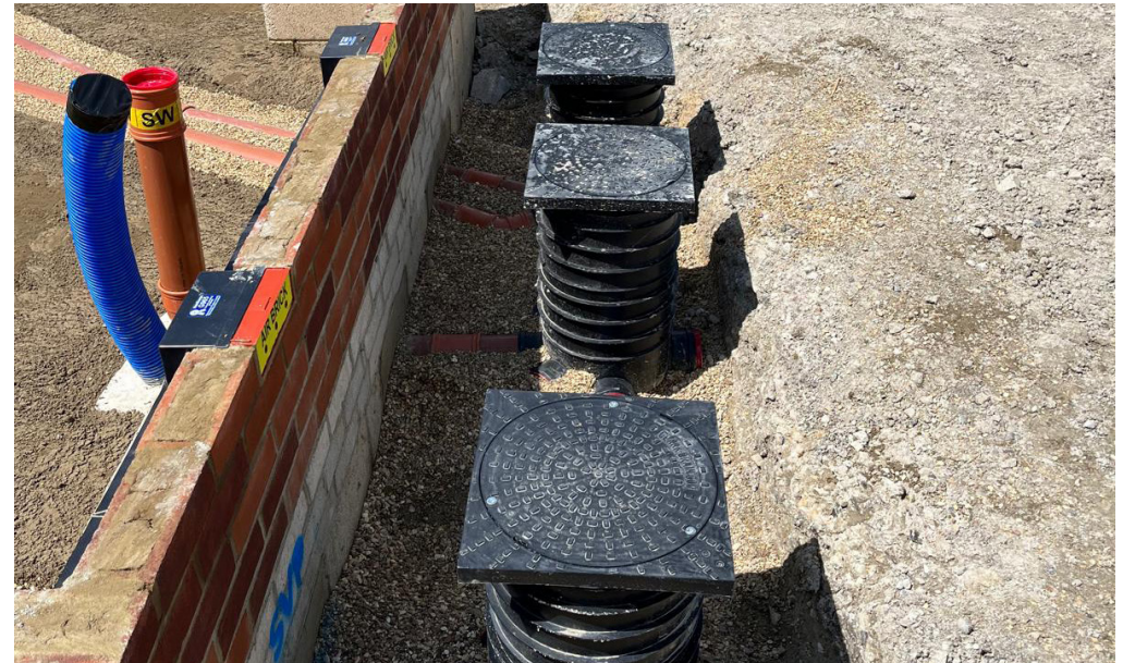
Inspection chambers have been positioned externally to ensure they align with landscaping and footpath details. Excavation work to accommodate drainage and bedding being laid is neat, straight and has uniform widths which allows alignment of the inspection chambers. Prior to backfilling of drain excavation all construction debris should be removed.
