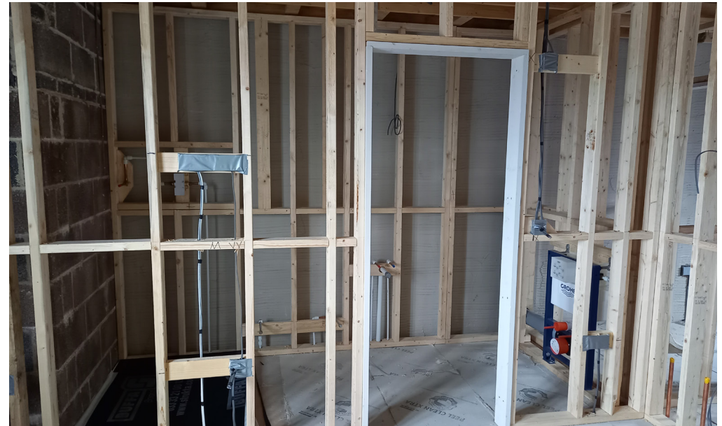
A well constructed timber stud work wall with studs accurately spaced, aligned, plumbed and levelled. Appropriate horizontal nogging has been set and electrical sockets supported by fixed grounds. An opening has been accurately formed for the door casing to be installed without excessive amounts of packing.
