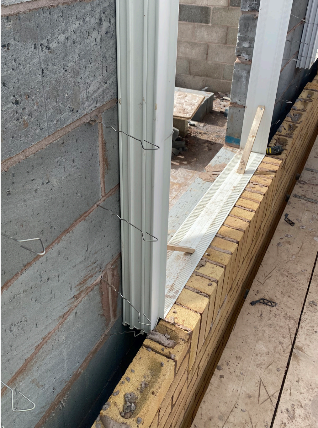
Reveal closure units being installed around an opening with an increased number of wall ties. Masonry has been struck clean and all joints filled with mortar. Closure units braced to ensure a square opening.
