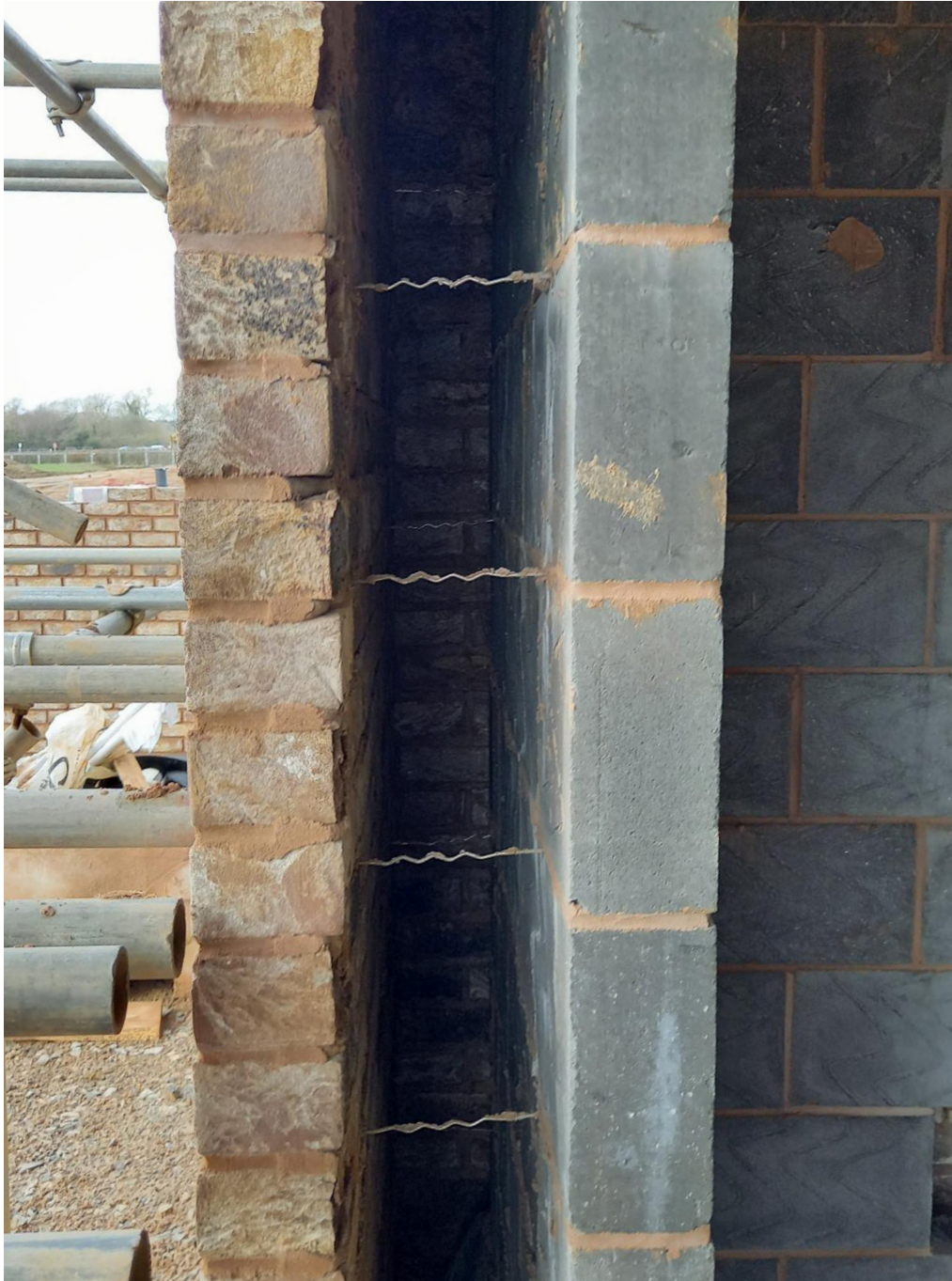
A masonry opening reveal with increased wall ties set to every block course. Wall ties are set to fall to the external leaf and now require removal of any residual mortar debris as part of the final preparation work.
