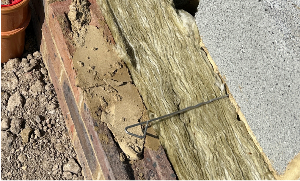
Insulation fully filling the substructure cavity and wall ties achieving correct embedment dimensions ready for placement of mortar.
