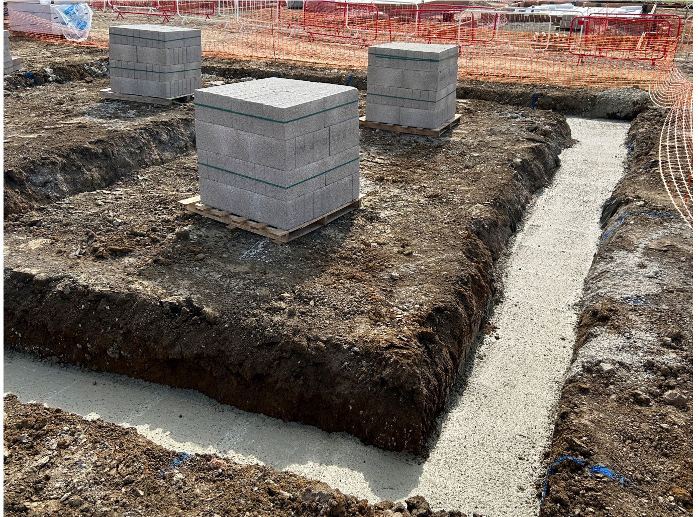
A level and organised area ready to start substructure masonry work.
