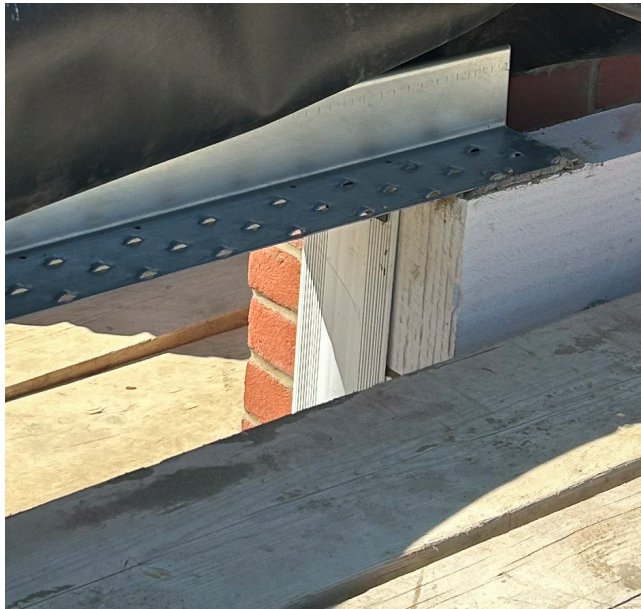
A steel lintel placed over an opening – end bearings are the required 150mm, and the lintel is fully bedded in mortar onto a full block masonry unit.
