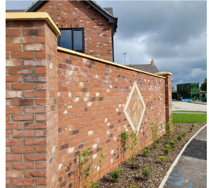
Neat detailing to the coping stones and well blended masonry units in this free-standing wall.
