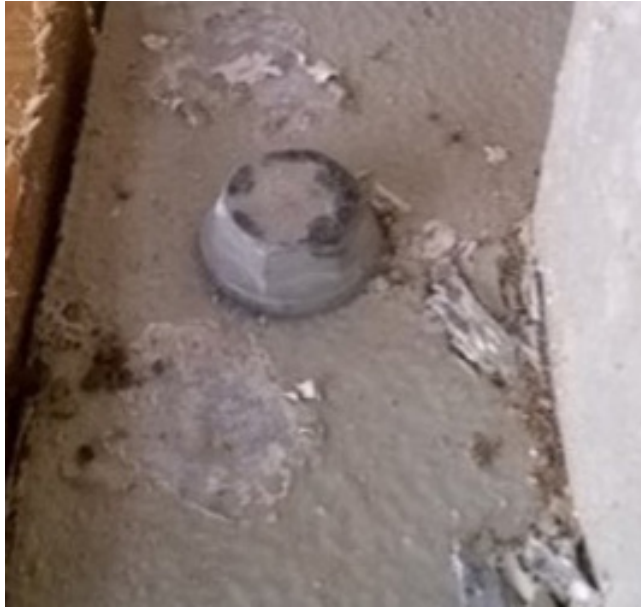
A fully fixed downwind post baseplate.
