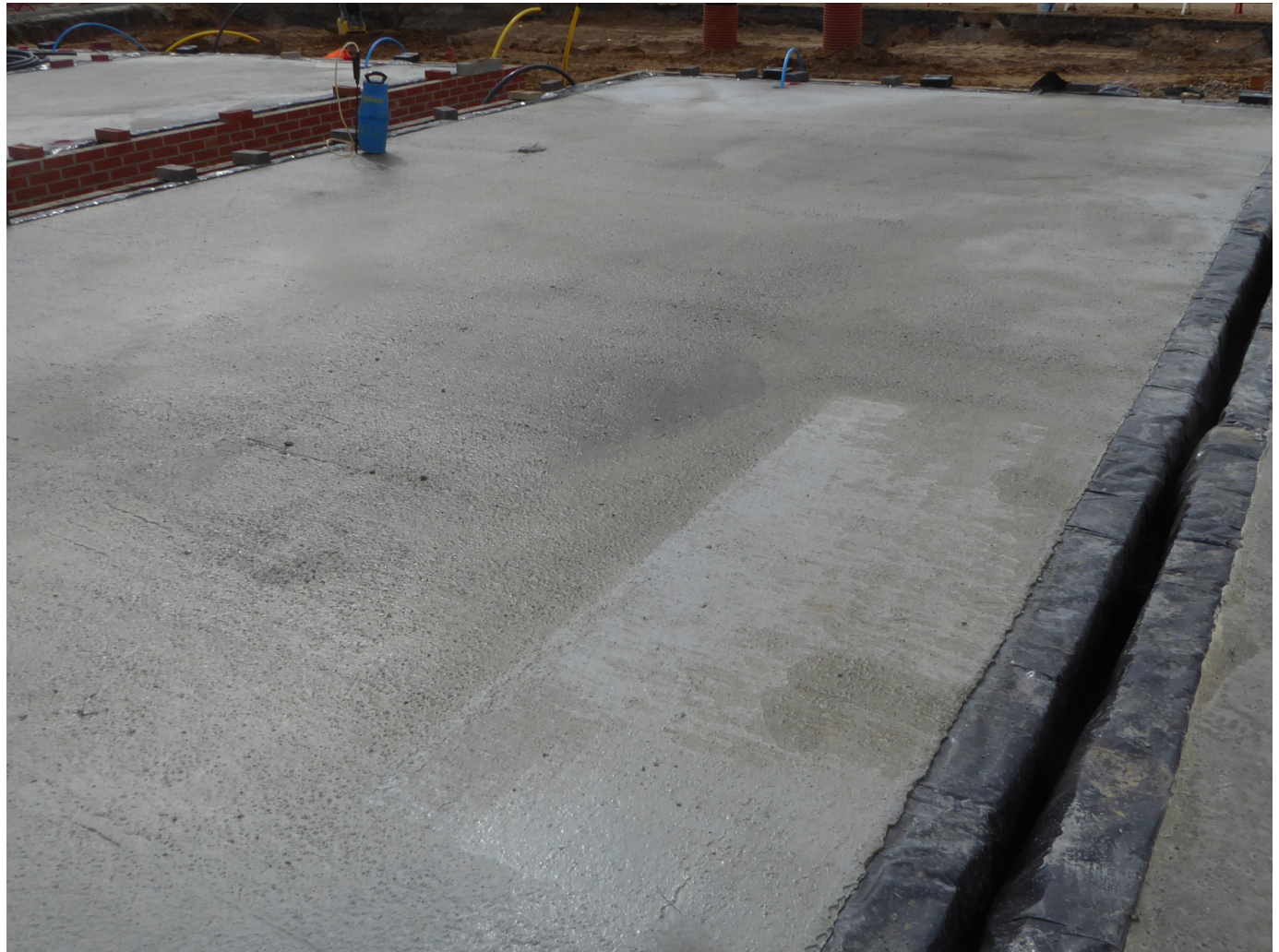
A completed concrete screed exhibiting a level and well finished surface. Edges are cleaned off, avoiding the need for mechanical removal of any excess material which can damage the membrane.
