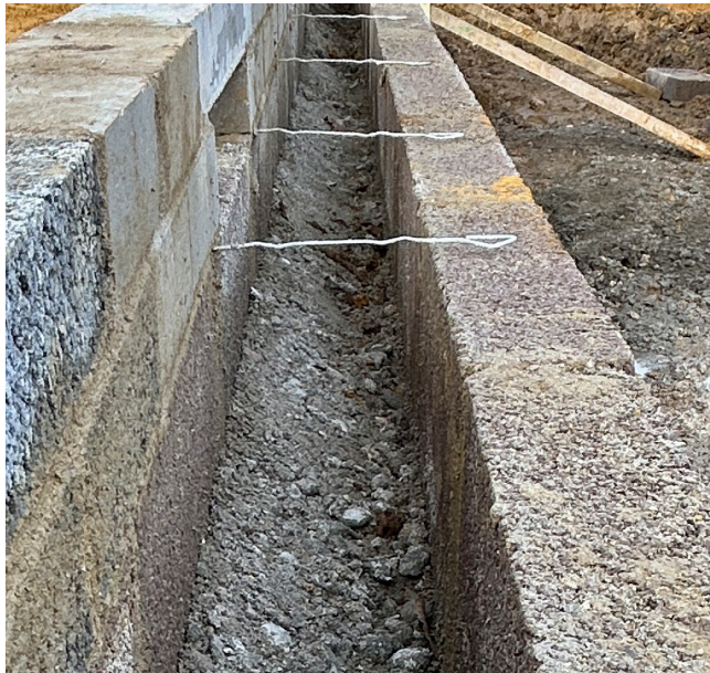
Clean cavity to external wall with lean mix set at 225mm below lowest DPC and set to fall to outside leaf.
