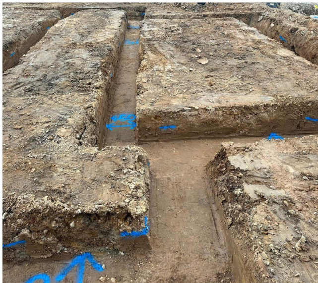
Excavation ready for concreting works to start. Demarcation for concrete levels marked on the sides of the excavation.
