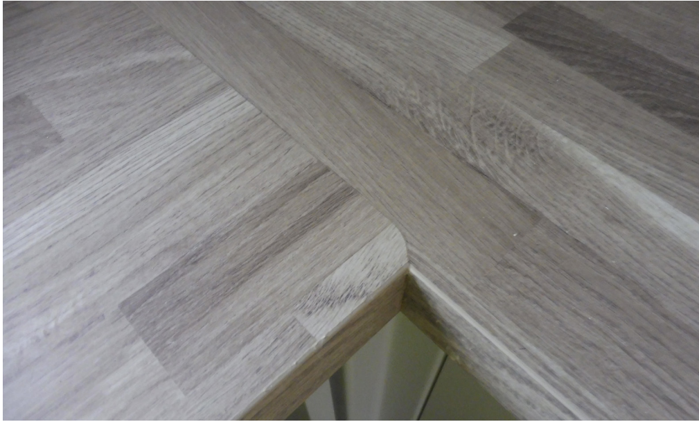
Neat, well executed finish work – butt and scribe joint to the worktop accurately completed.
