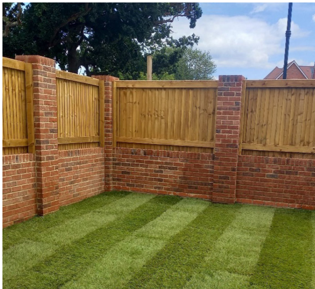
A brick and timber panel boundary wall. Masonry is well executed with clean detailing to the brick capping details. Timber panel work is neat, level and even all around.
