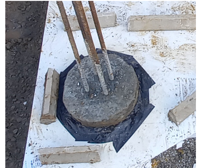
Post casting, the piles have been carefully cut down to the required level. The top surface is prepped, and work has been completed to seal around the pile heads. Spacers to support the reinforcement in the follow-on construction are in the process of being placed.
