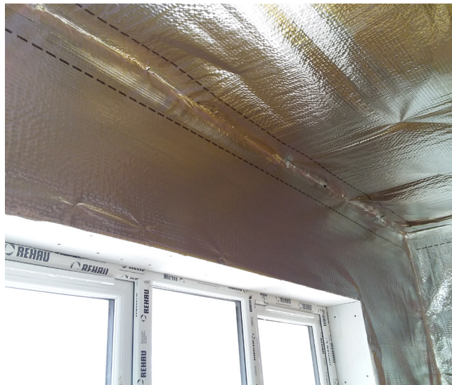
An Air and Vapour Control layer installation executed to achieve continuity around junctions with the ceiling and around internal corners.
