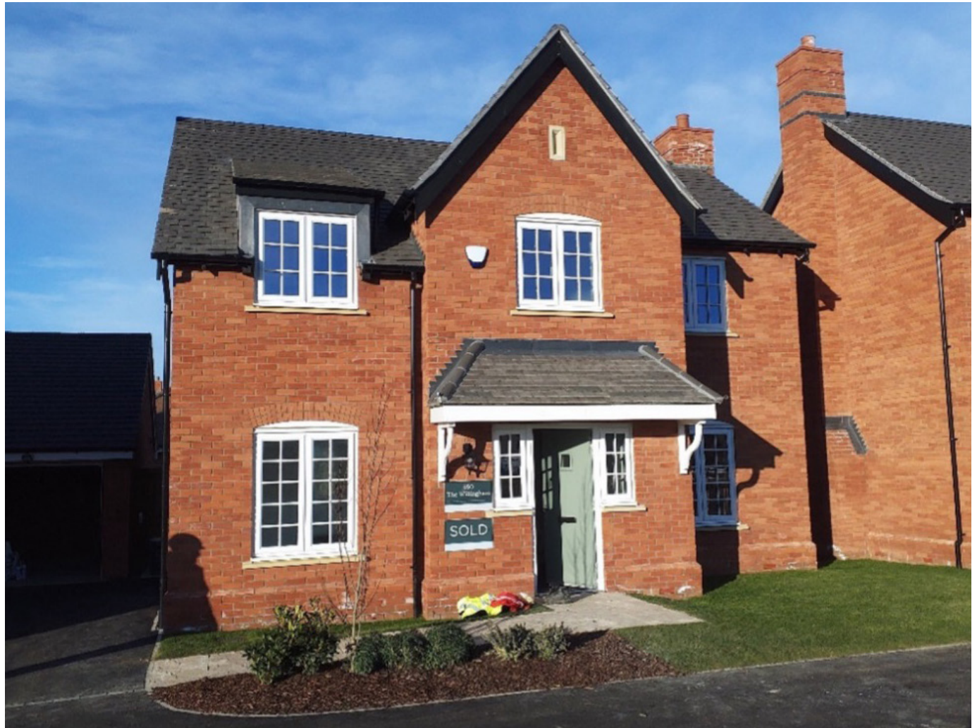
A well presented façade - free from excessive mortar smears, staining, or discolouration that detracts from the overall appearance.
