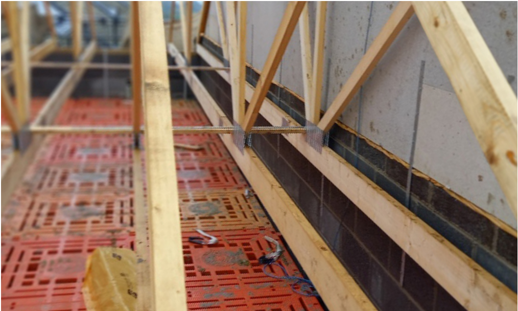
Vertical proprietary metal straps correctly fixed through into stud locations within this spandrel panel and into the blockwork below. Longitudinal bracing is tightly abutting the face of the spandrel and further secured with restraint straps.
