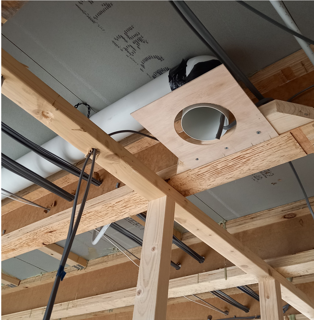
A timber truss and ground used to accurately locate the duct. The mechanical fan outlet has also been provided with a robust fixing position during 2 nd fix.
