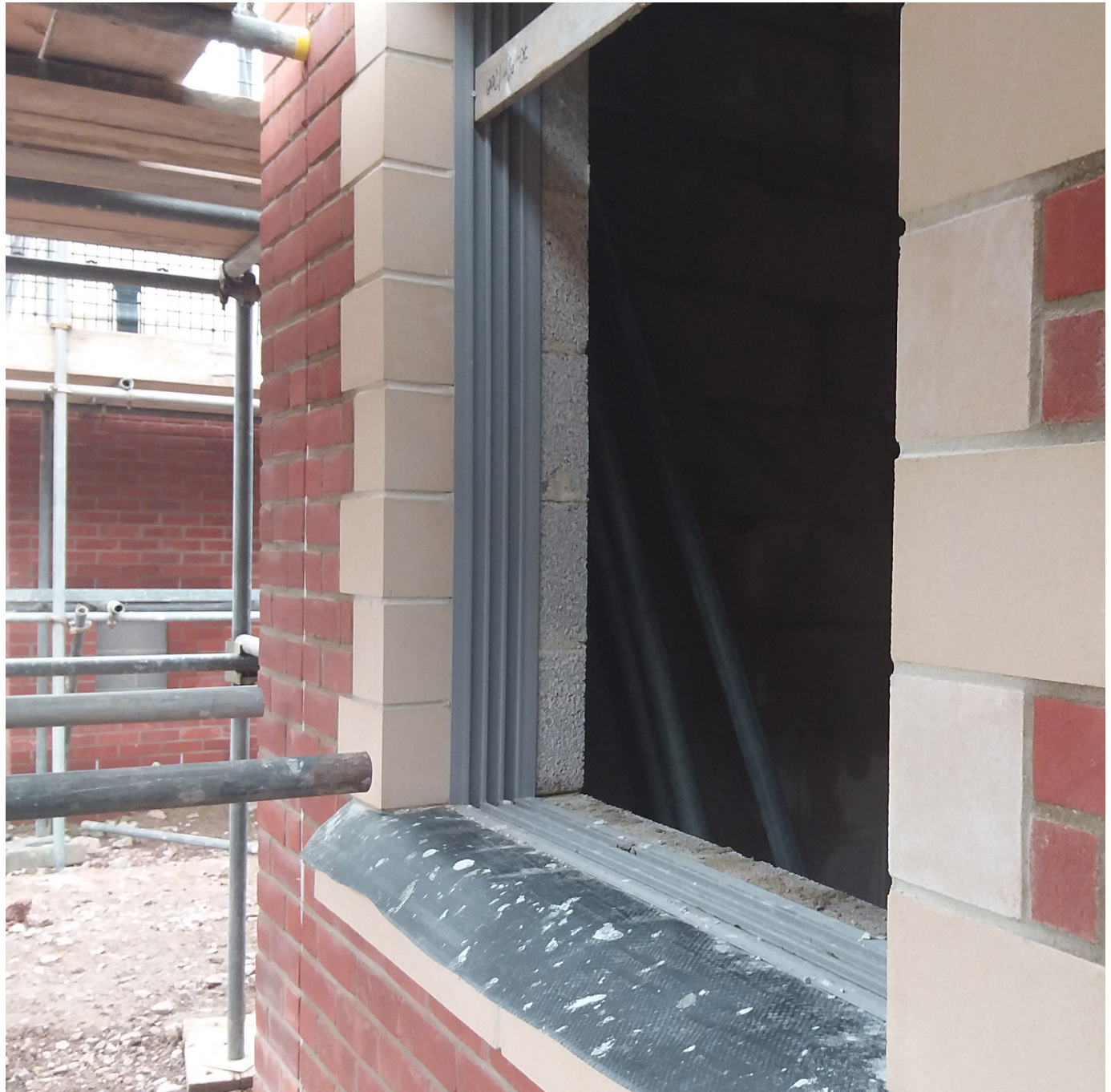
Architectural feature stonework completed to a high standard around this window opening. Joints between units are uniform and stone faces are extremely clean. Protection has been built into the jambs to protect the stone sill from mortar deposits. This can be neatly trimmed off when masonry works are completed.
