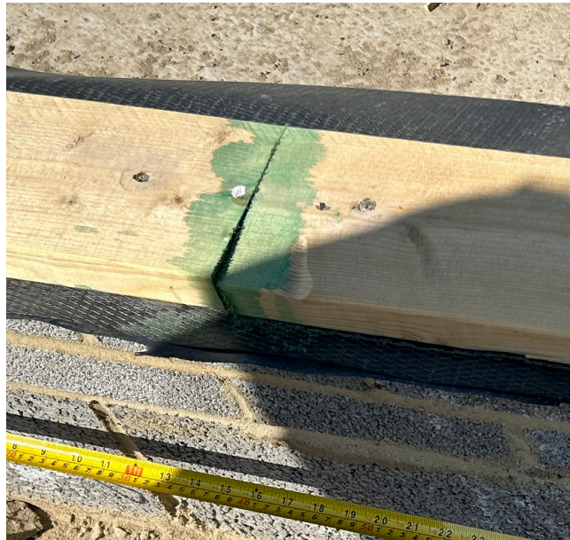
Sole plate cut ends correctly treated with preservative to protect the timber end grain.
