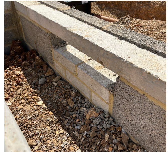
Lintel placement for a telescopic ventilation penetration into a sub-floor. Oversizing the opening allows for adjustment to fit in with coursing in the external splash course.
