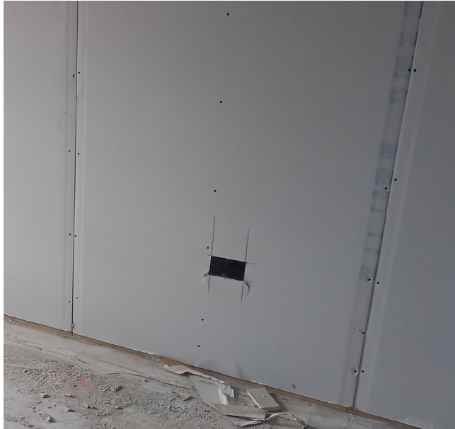
Uniform and correctly spaced screws securing the wall plaster boarding. Board joints are nominally 3mm in width. Cut out work around socket is neat and square.
