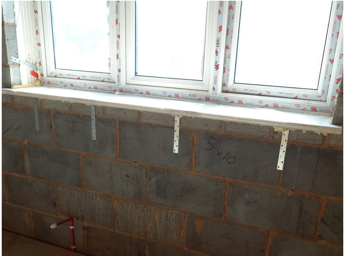
Equally set steel angle brackets fixed to the underside of this window board and then secured to the masonry below. Expanding foam has been used in between fixed points to offer additional fixity.
