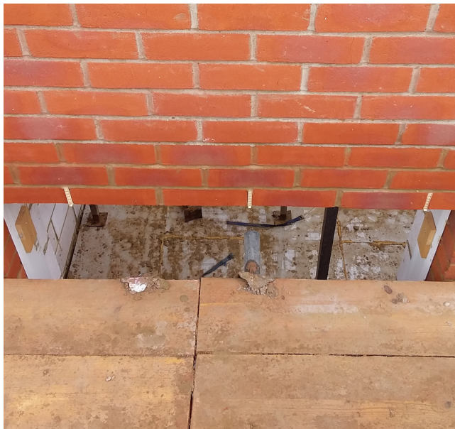
Masonry completed at this lintel position, weep vents have been uniformly spaced to both drain and ventilate the cavity which is essential for timber frame construction.
