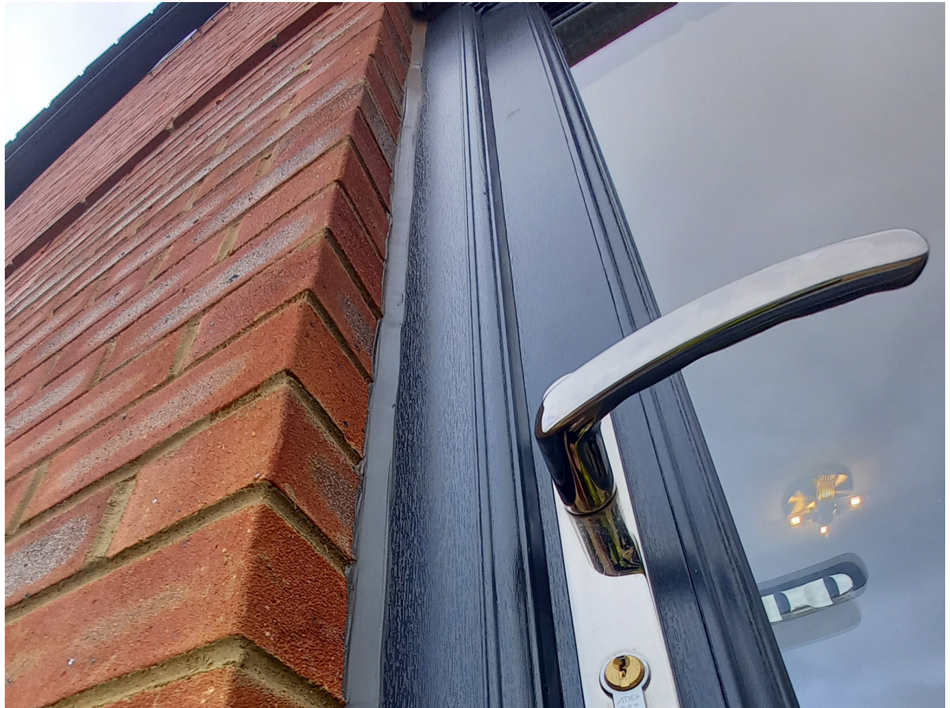
A continuous seal of the perimeter joint to this door. Sealant is well tooled and free from gaps and smears.
