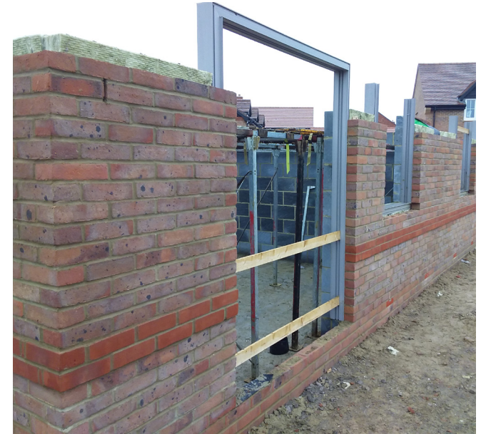
Proprietary thermal cavity closure units being built into openings. Bracings have been applied at corners and across the openings to ensure they maintain an accurate shape.
