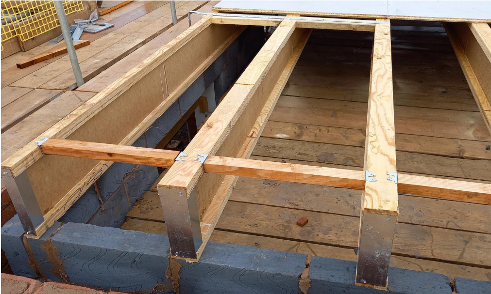
Engineered I-joists with a full end bearing onto masonry. Metal end caps have been attached to protect and stiffen end bearing. These caps also facilitate neat and tight masonry placement around end bearings. Joists also incorporate tightly fitted strutting to reduce risks of rotation.
