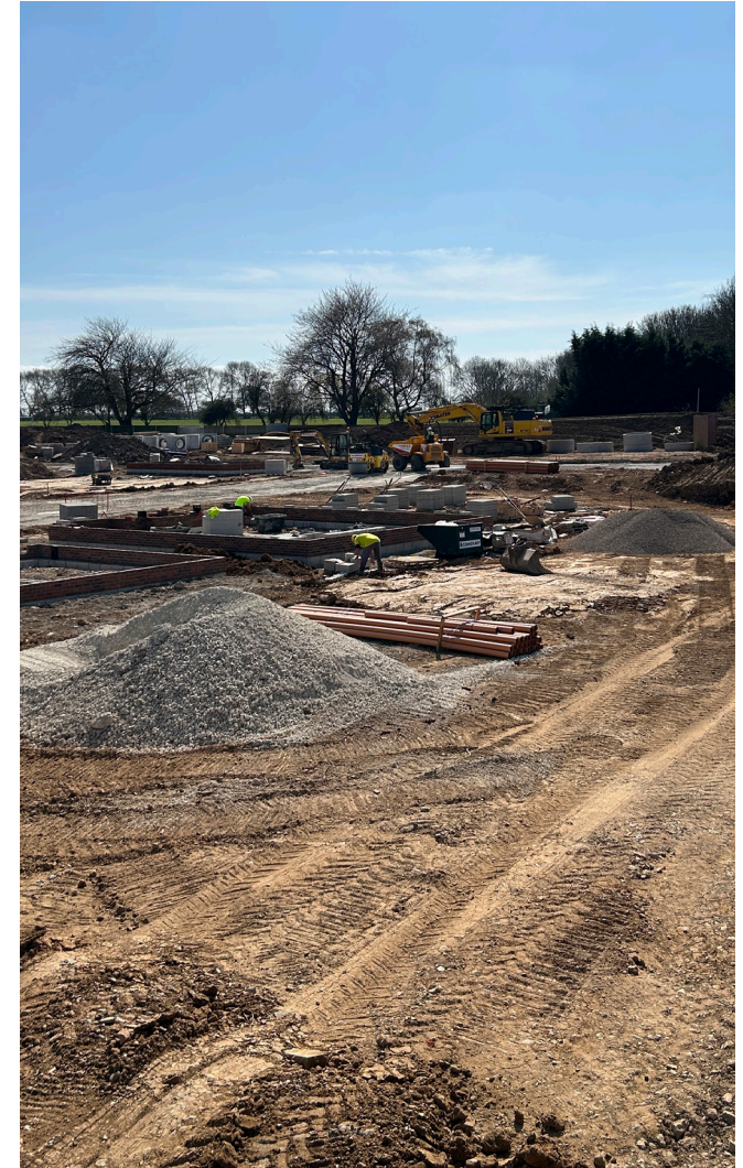
Clear segregation of excavated soils from crushed stone aggregates to avoid risks of mixing materials.
