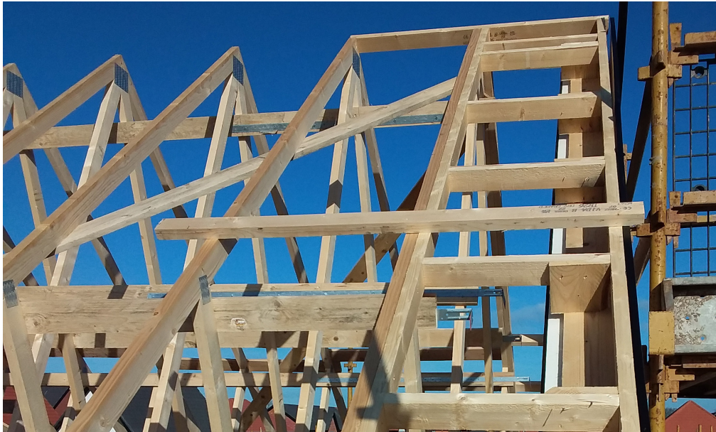
A ladder frame construction fixed to the last trussed rafter. Its height location and level are set off adjacent trussed rafter backs using temporary horizontal timber bracing. Additional solid blocking has then been introduced and squarely fixed into the ladder frame and the head of the timber spandrel.
