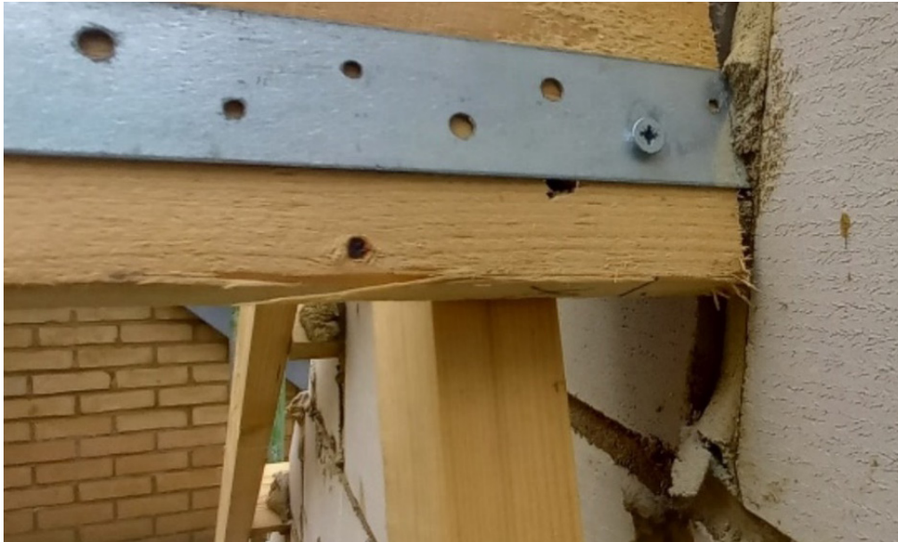
This arrangement has the lateral restraint fixed onto the longitudinal brace. The strap has been neatly located through a perpendicular mortar joint and 'hooked' within the cavity at a full block.
