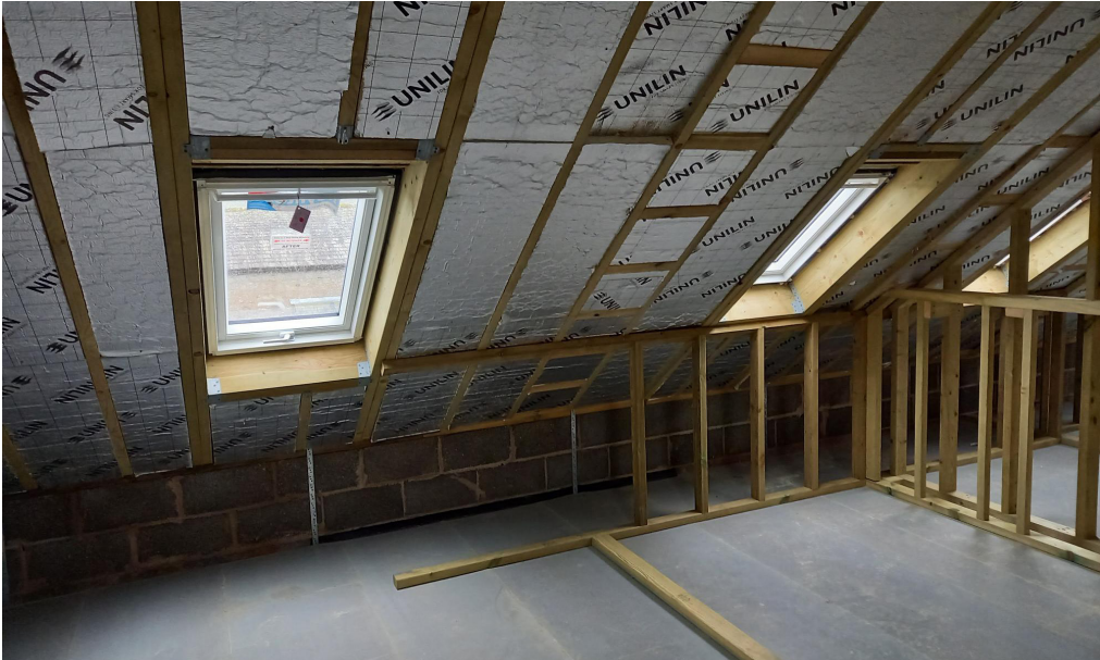
Rigid insulation installed in between rafters in a pitched roof. Cutting of the board has been completed accurately to be tightly friction fit.
