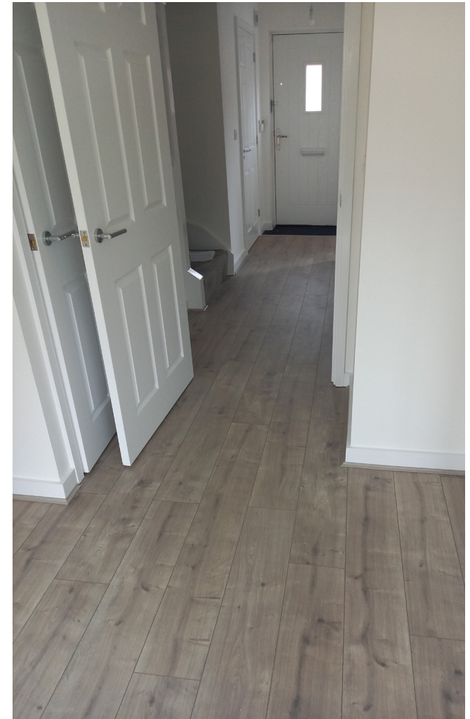
Flooring laid with straight even joints. Edge detailing in this example has been completed with neat scotia trim with neat and well executed jointing.
