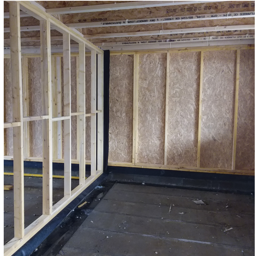
Ground floor timber frame panels erected. DPC material projects from the base and either side of the internal wall location to facilitate connection with AVCL.
