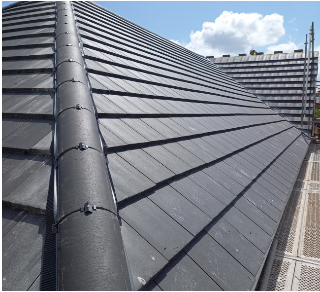
A well-executed installation of a proprietary dry hip fixing system. The ventilated hip roll is neat and uniformly laid and each tile union is well fixed with a union seal and fixing plate.
