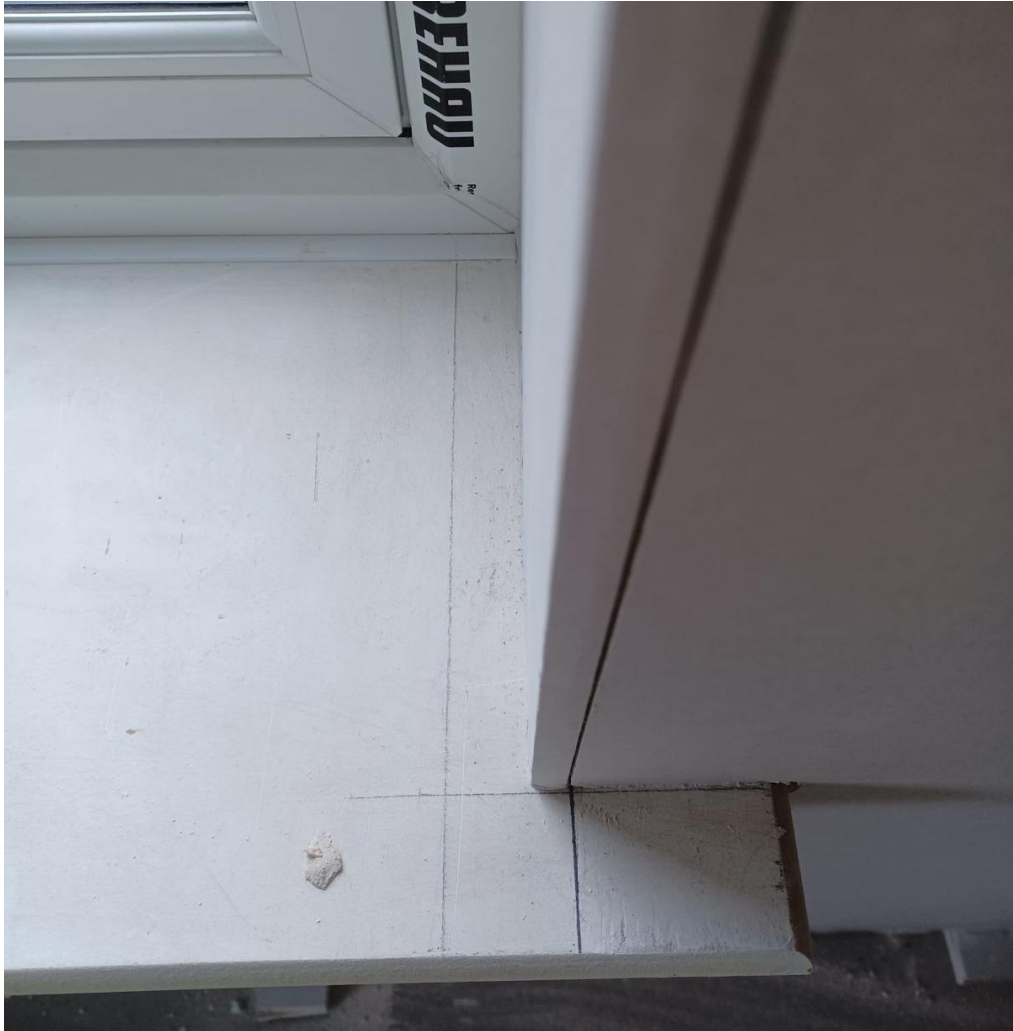
Well presented plaster board reveals with plumb and square board application, achieving equal margins to window jambs. Board termination under window board is neat and the gap is not excessive.
