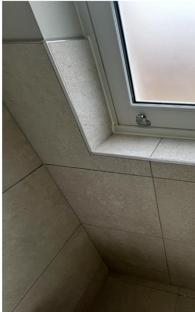
Cut tiles to this window area have been neatly cut and completed with edge and corner trims.
