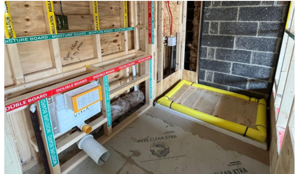
Excellent levels of preparation for plaster boarding works with demarcation tapes being used to ensure correct board specification is followed.
