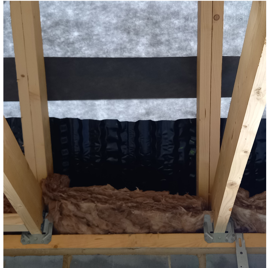
A proprietary eaves panel vent installed to ensure the cold pitched roof is appropriately ventilated. A portion of insulation has been installed neatly behind the wall plate whilst this area is accessible from the underside, ensuring continuity is achieved with the cavity wall insulation and behind the timber wall plate.
