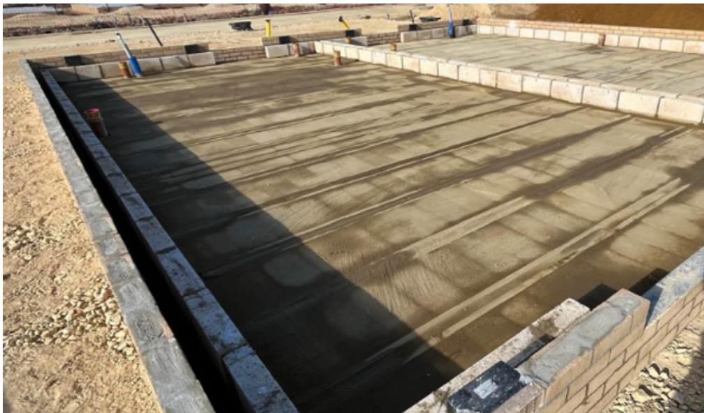
Slurry coat brushed into the beam and block floor construction, filling all joints.
