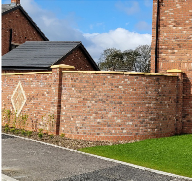
A well executed curved freestanding wall with neat coursing and jointing.
