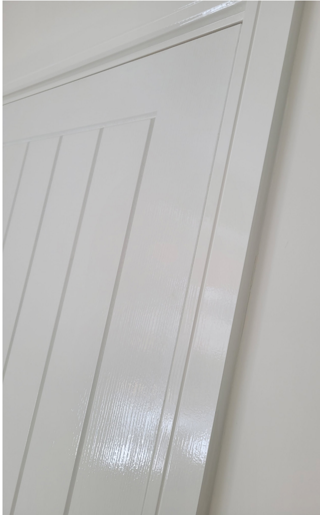
Internal woodwork finish free from brush and roller marks.
