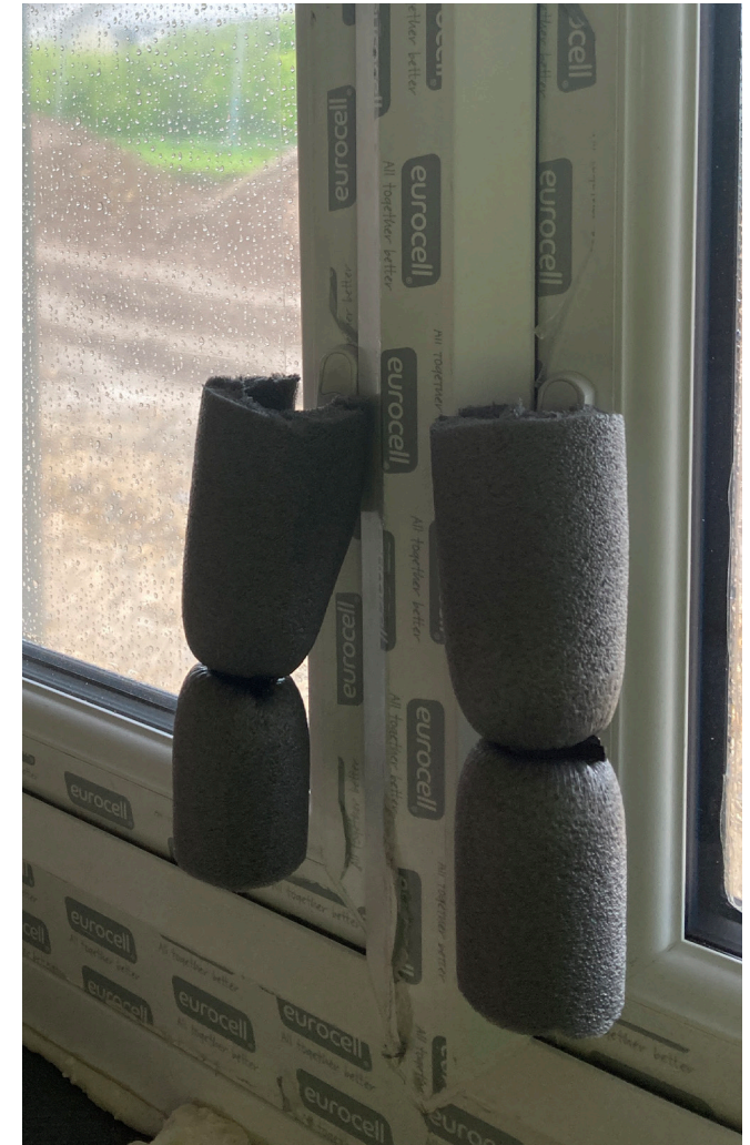
Protection to handles being utilised from the outset to avoid damage from follow on construction operations.
