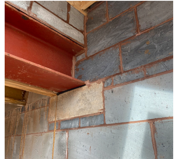
A large structural beam bearing onto a concrete padstone. Great attention has been paid to completed masonry around the beam end with neat mortar pointing.
