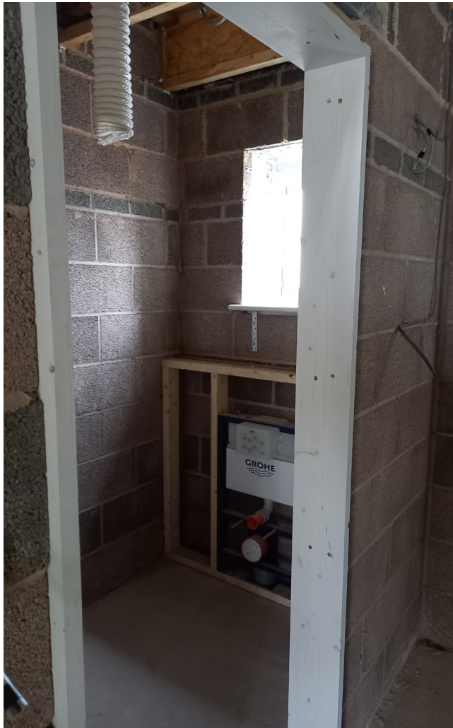
An example of paired fixings to the jambs of a door casing to fully secure the frame into the surrounding substrate.
