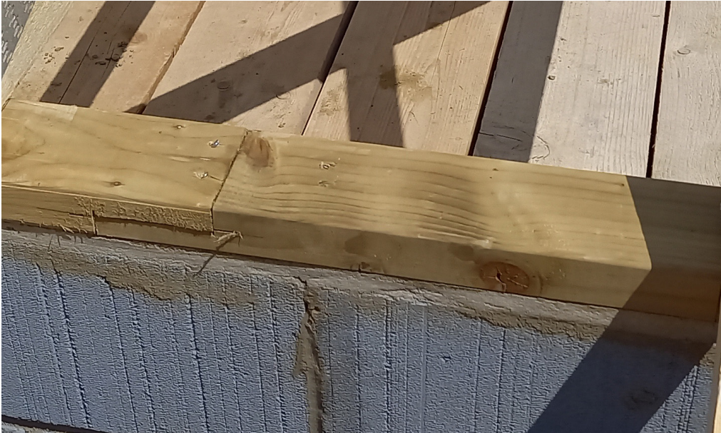
A wall plate bedded level, with the running joint half-lapped and nailed.
