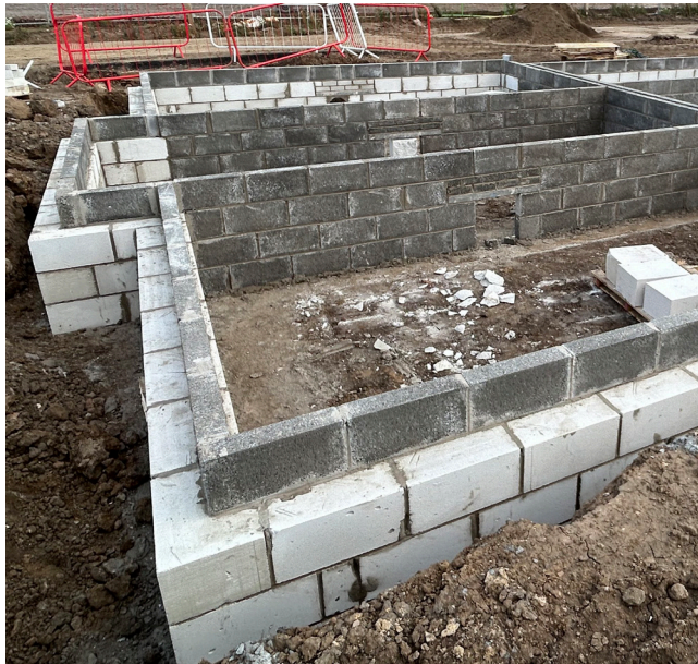
Clean work area with well executed laying of trench block and concrete blockwork. All joints filled with mortar and neatly struck.
