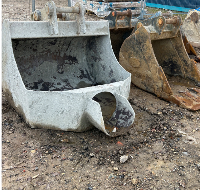
Concreting chute bucket ready to be attached to assist in a controlled delivery of concrete into the excavation.
