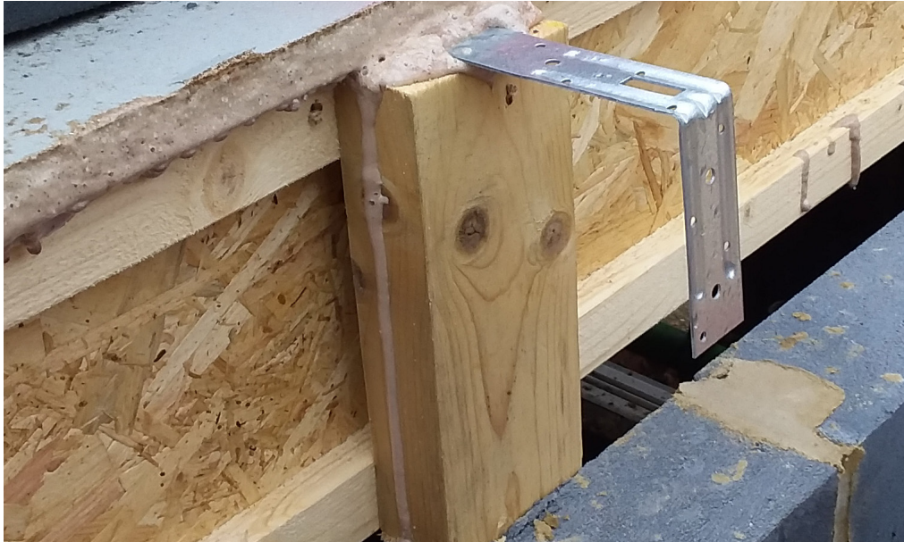
Final blocking piece between masonry set and fixed. Lateral restraint strap is now set and ready for masonry work.
