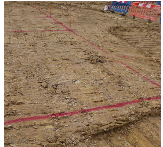
Planning and marking out for accuracy in the excavation formation.
