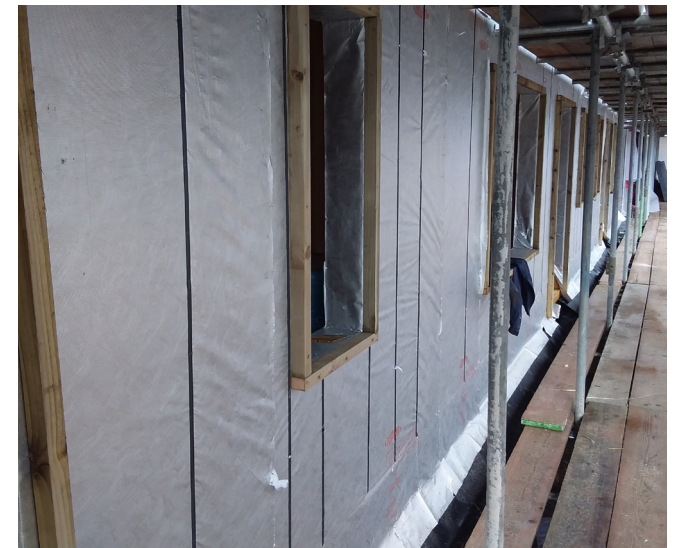
External breathable membrane work carried out to a good standard. Membrane work within opening reveals is continuous and sealed with the internal AVCL. Demarcation taping to stud positions is consistent for wall tie placement and overlapping with the cavity tray at low level has been completed.
