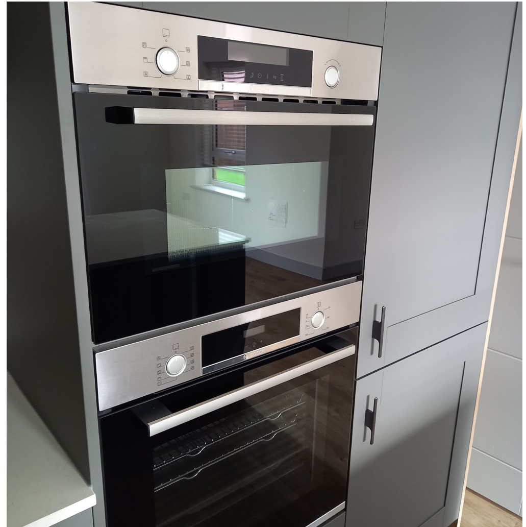
All integrated appliances should be securely fitted and level to prevent movement or vibration. Appliance doors should align flush with adjacent units, panels and doors to provide a neat finish.
