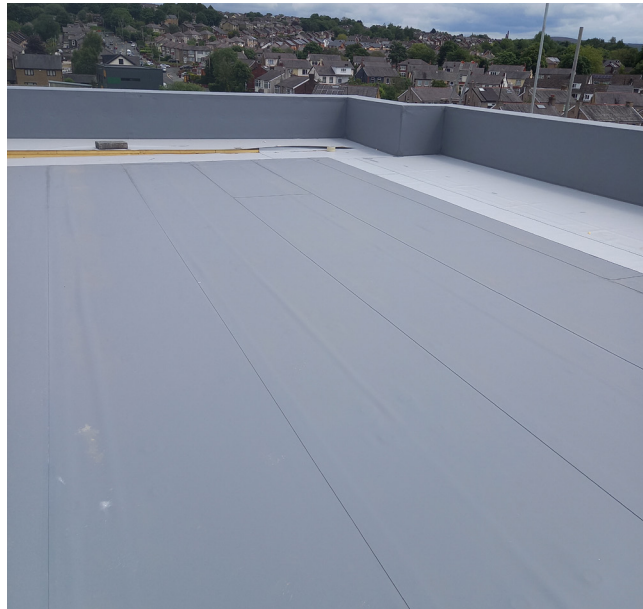
Work on going to a single ply flat roof installation. Parapets are fully encapsulated with the roof covering material returning onto the head of the parapet wall.
