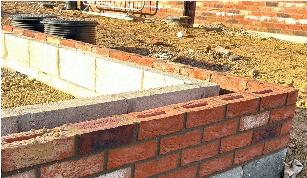
Well executed facework in this splash course masonry. Joints are fully filled and have consistency in relation to their size between masonry units.
