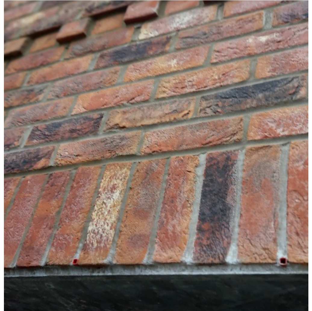
Neat masonry facework above an opening complete with weep holes. Weep holes are clear from mortar and slightly pronounced.
