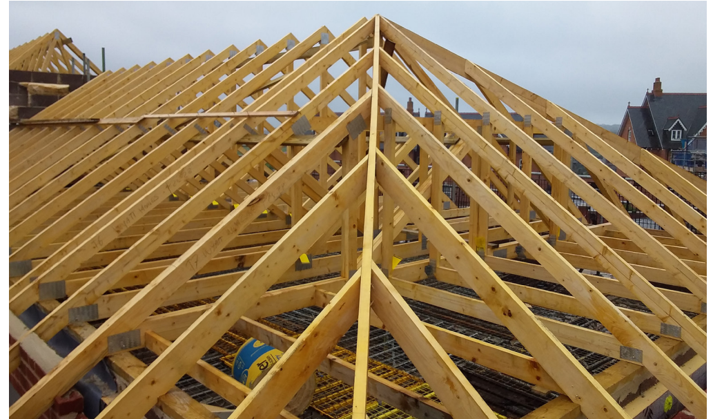
A hip to a trussed rafter roof securely fixed to the trusses at appropriate intervals with good alignment and level, giving support and stability to the roof structure.
