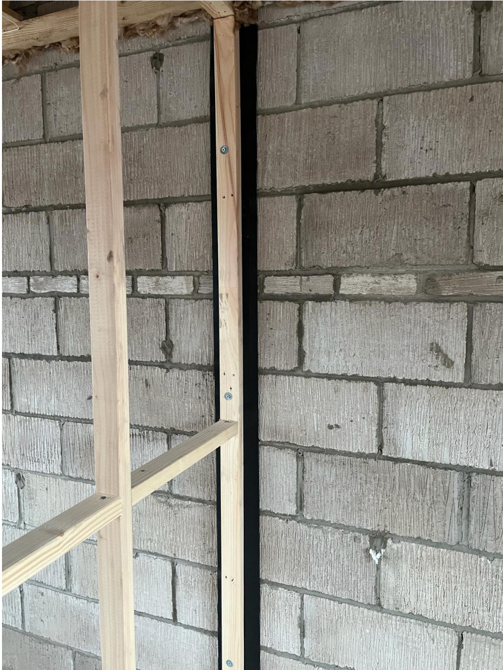
The fixing of stud work into the masonry structure. Shot fired nails have been used to set plumb and then screwed fixings have been employed to secure the stud work. Steel washers have been used in this instance to ensure the screwed fixings achieve maximum fixity.
