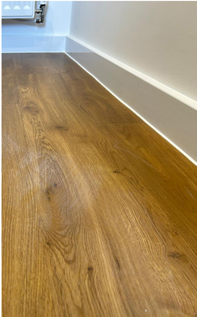
Edges where flooring meets walls, skirting, or other surfaces should be cleanly cut and sealed.
