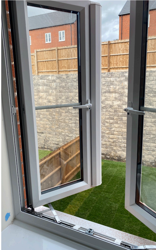
A window installation undergoing final checks – hinges, operation and locking mechanisms should be verified by the installer to satisfactory performance in terms of security, weathertightness, and exclusion of draughts.
