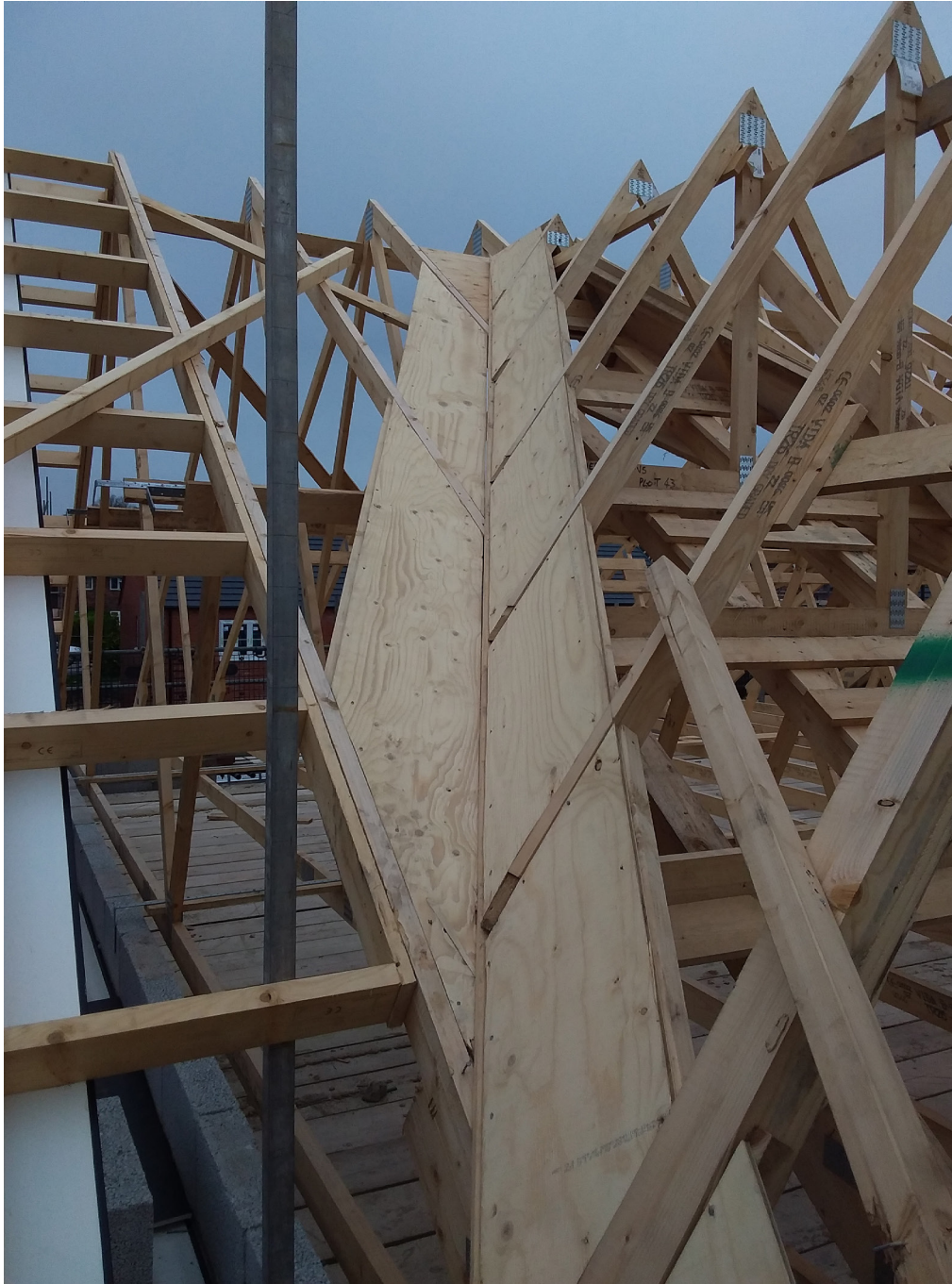
A ply valley board on a trussed rafter roof, secured and set to finish level with the upper surface of the rafter backs. Additional noggings have been fixed to support valley edges providing a solid base for the placement of the follow-on roof covering work.
