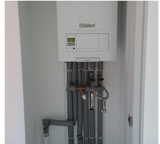
Exposed pipe work in these heating appliance cupboards has been fully insulated. Insulation material secured with cable ties and all joints neatly formed.
