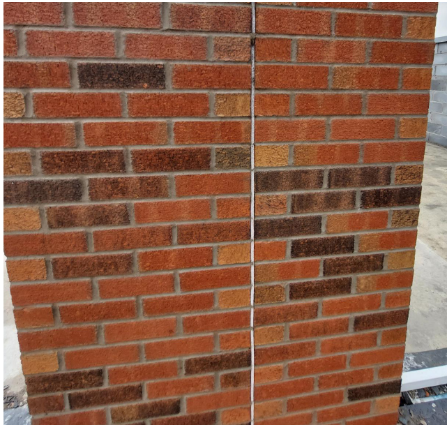
A neatly constructed masonry panel with a centrally located movement joint. Compressible polyurethane foam has been placed during construction to facilitate joint sealant application.
