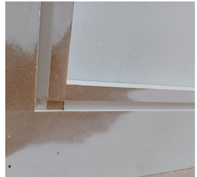
Skirting board with tight mitred external corners and internal corners accurately scribed to suit the section profile.
