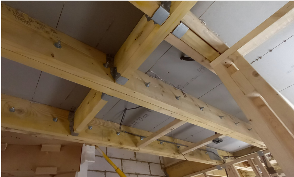
Bolted solid timber joists have been connected here to create a stronger, more stable built-up beam arrangement. Bolted connections have been well executed, with a uniform linear pattern down the centre line.
