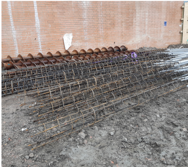
Reinforcement cages – fabricated as per the engineer's details, complete with protective material to uppermost ends.
