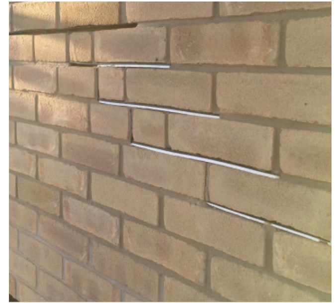
The position of the cavity tray has been clearly determined. A horizontal raked joint and small widths of removable material have been placed 25mm into the masonry, under the leading edge of the cavity tray in the stepping mortar beds ready to be removed and receive the abutting roof flashings.
