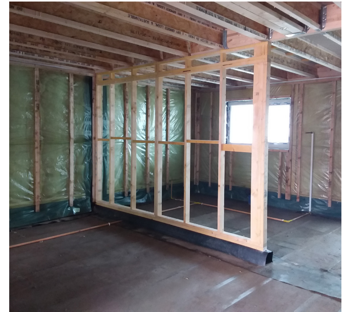
Clear Air and Vapour Control layer installation work executed to a good level. Sealed onto the projecting DPC at the base and vertical DPC at the internal wall union. Counter batten work employed to facilitate placement of follow-on services without the need to penetrate the AVCL.
