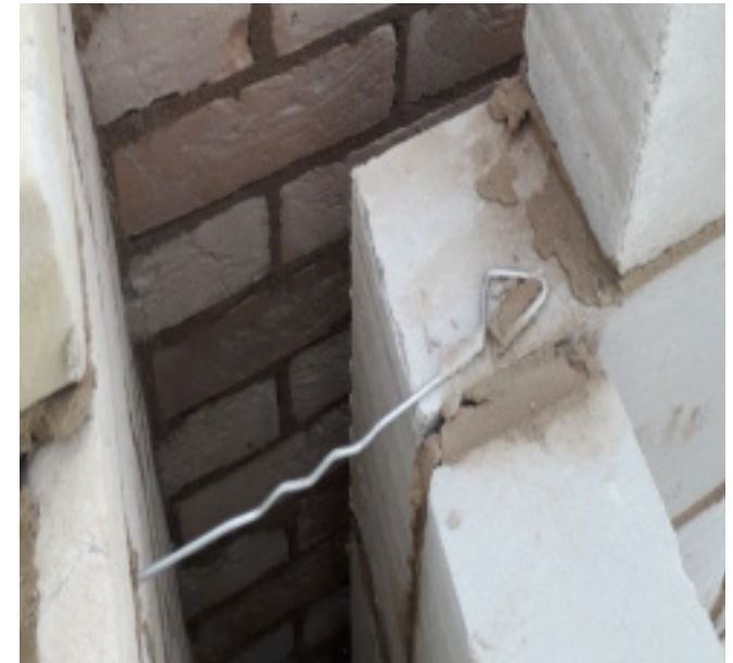
Wall tie placement achieving the required minimum embedment dimension and displaying a fall from inside to outside. Cavity is clean, with all joints fully filled and struck.
