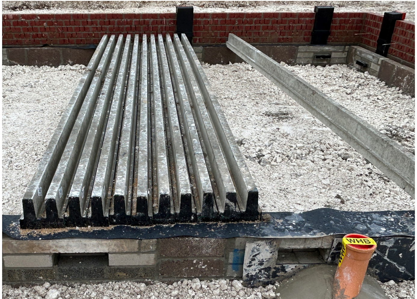
Beams have been temporarily placed onto substructure masonry at the plot to elevate off the ground. Extra precautions for material protection with beam ends painted with a protective coating.
