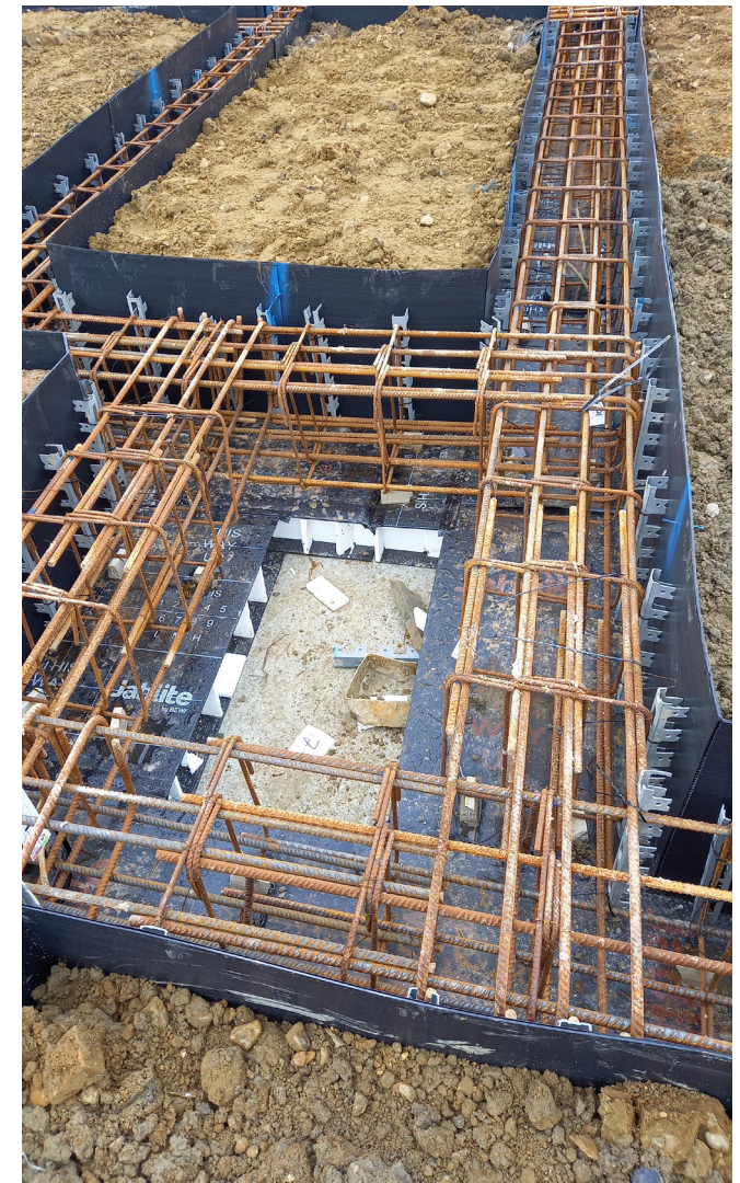
Ground beams being laid over void formers. Bars are tied and lapped. Formwork is well constructed to give the required support to concrete placement work.
