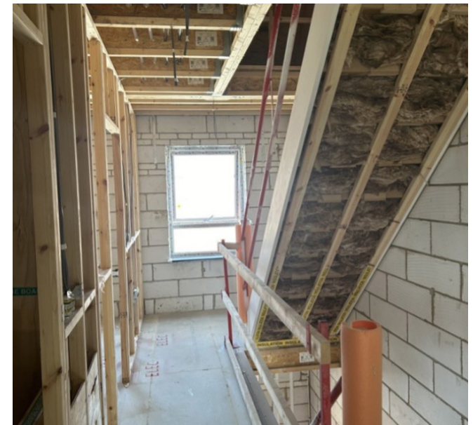
A straight flight installed with acoustic insulation to reduce noise transfer, secured in place prior to plaster boarding.
