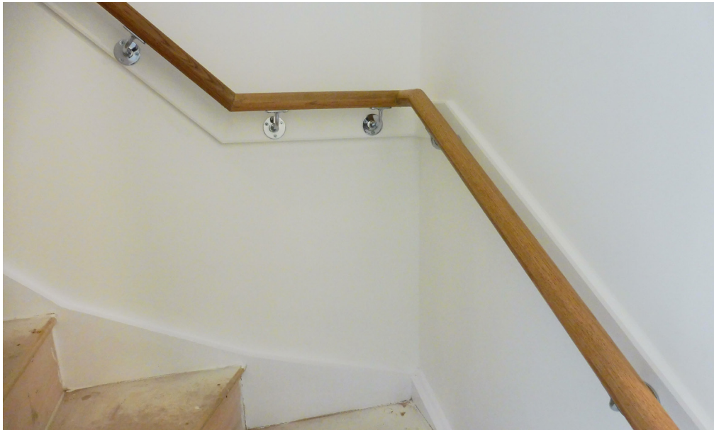
A well executed handrail installation – multiple changes of direction and angles have been neatly formed.
