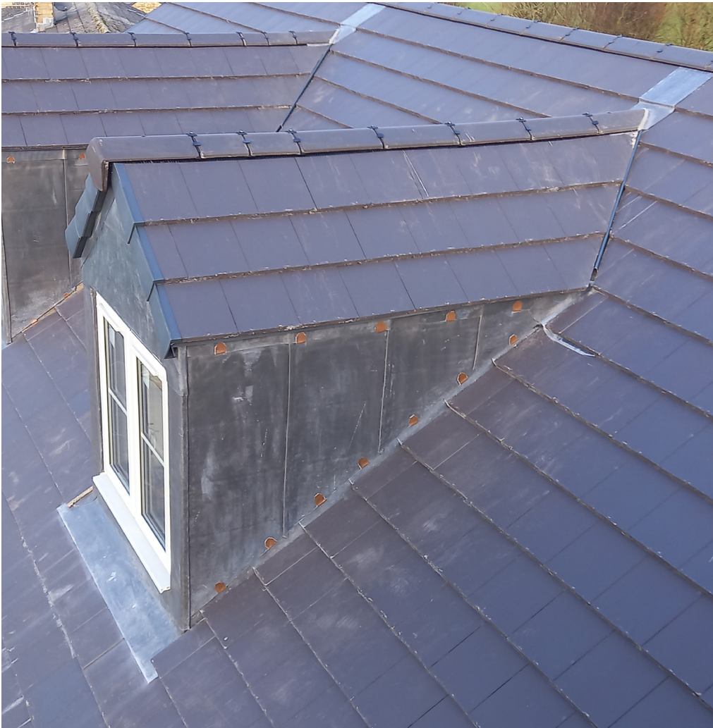
Lead work completed to this dormer construction – corner welts have been formed correctly with the forward-facing jamb side dressed around to finish onto the dormer cheek. Joints are secured down with welted joints. Edge clips have been fixed at uniform centres.
