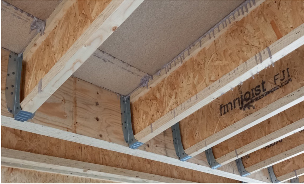
Engineered I-joists fully seated and fixed into metal hangers onto an engineered timber beam. All nailing has been completed to the beam and the I- joists.
