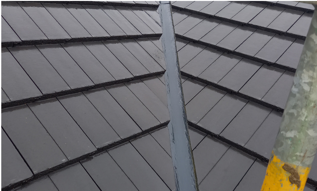
A neatly installed open preformed valley. Tile lines are well aligned and cutting work neat and tidy.
