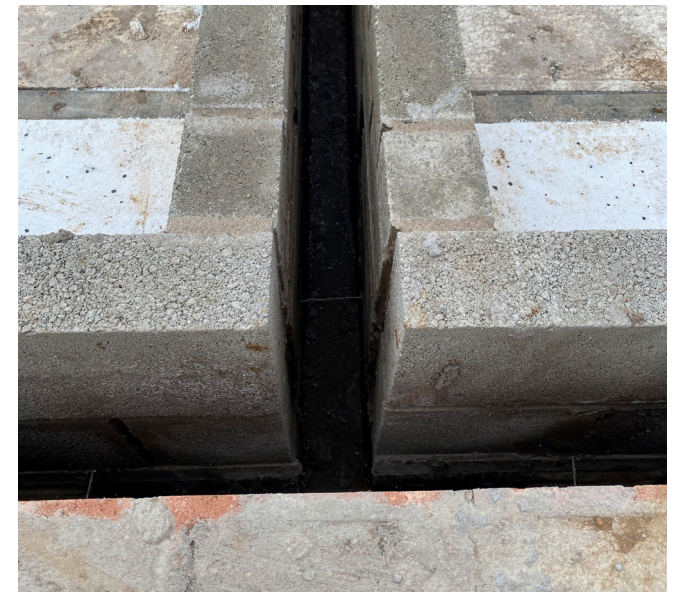
Coursing blocks laid to a high standard of workmanship, fully supported, and bedded in mortar with perpendicular joints fully filled. Cavities being kept clear and free from mortar.
