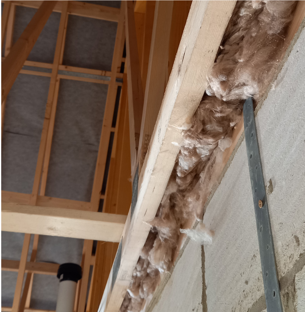
A portion of insulation has been installed in between the last trussed rafter bottom chord and base rail of the timber spandrel panel whilst this area is accessible from the underside. An example of good forward thinking to ensure continuity of the thermal envelope is maintained.
