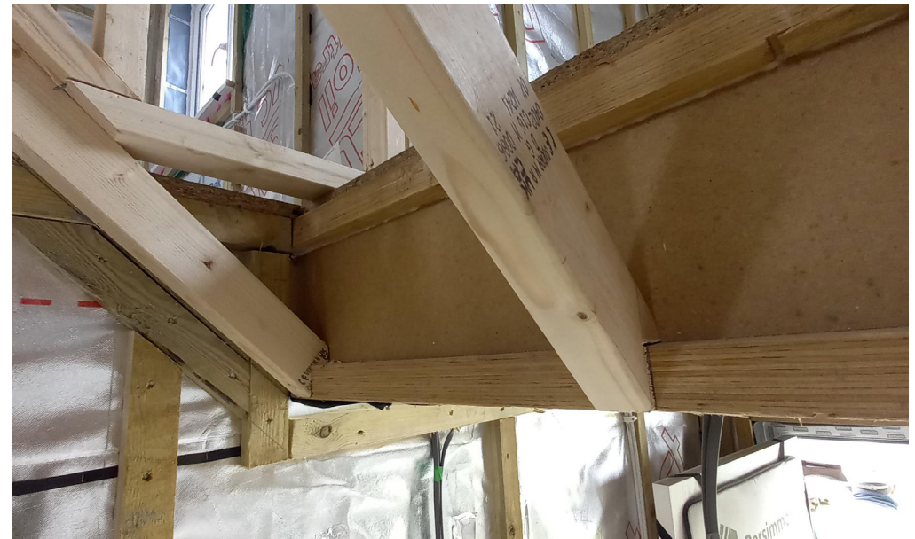
A staircase bulkhead boxing out with timber sections executed with precision with tight and flush fitting joints ready to receive plasterboards.
