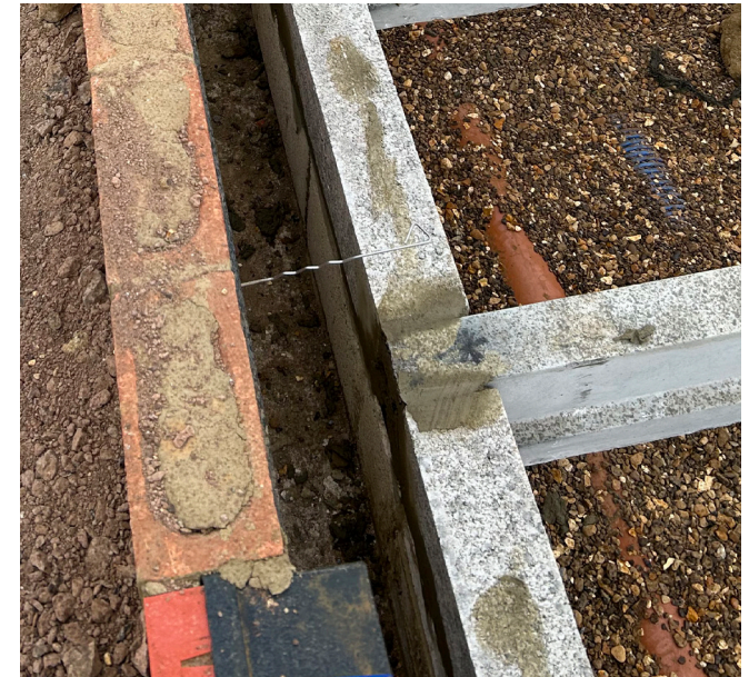
Beam spacer blocks fully bedded on mortar with fully filled joints to beam ends.
