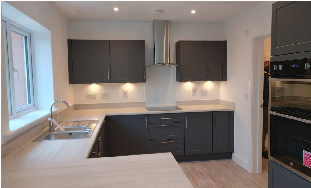
A well presented kitchen installation.
