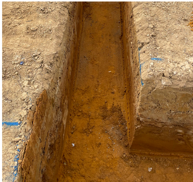
Foundation excavation with precise dimensions, a flat and level base and good verticality in the sides.
