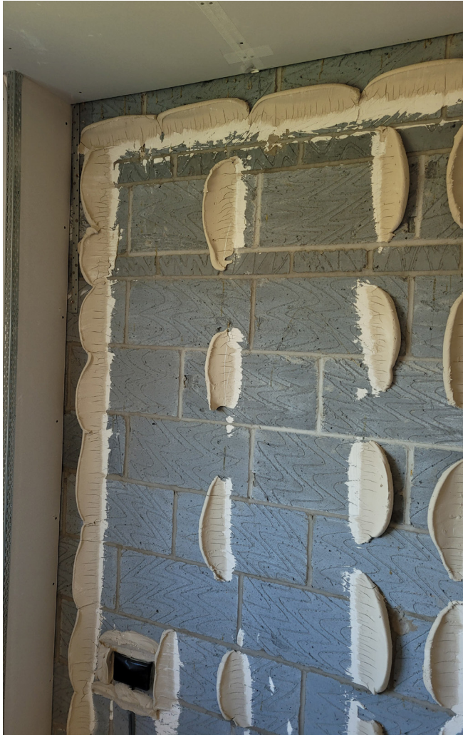
Evenly spaced adhesive dabs at 250mm long by 50mm. A continuous ribbon of adhesive has been used at wall perimeters and around the socket location.
