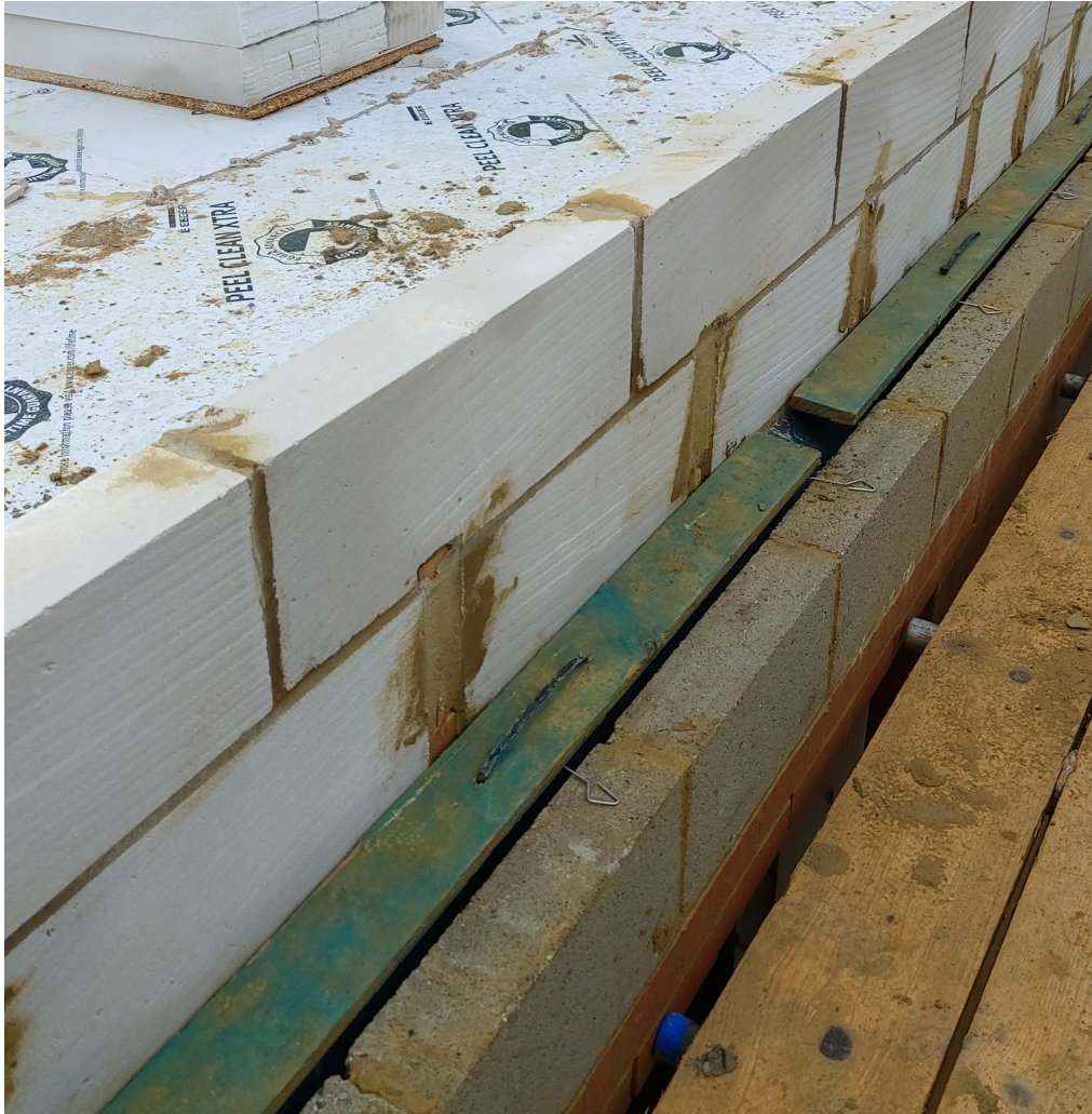
Larger sized masonry units have been installed to a good standard. Joints are fully filled and gaps around the intermediate floor joist ends have been fully pointed with mortar. A cavity lath is being used to control the risk of mortar debris dropping into the cavity below.
