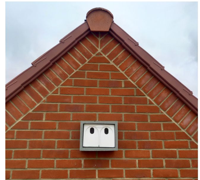
Verge masonry detailing has been well executed. All joints are neat, uniform in size and well finished. Cut units are precise and well aligned.
