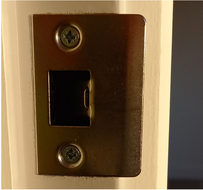
Great examples of well executed ironmongery installation – tightly fitted into accurate recesses, and free from scratches and damage.
