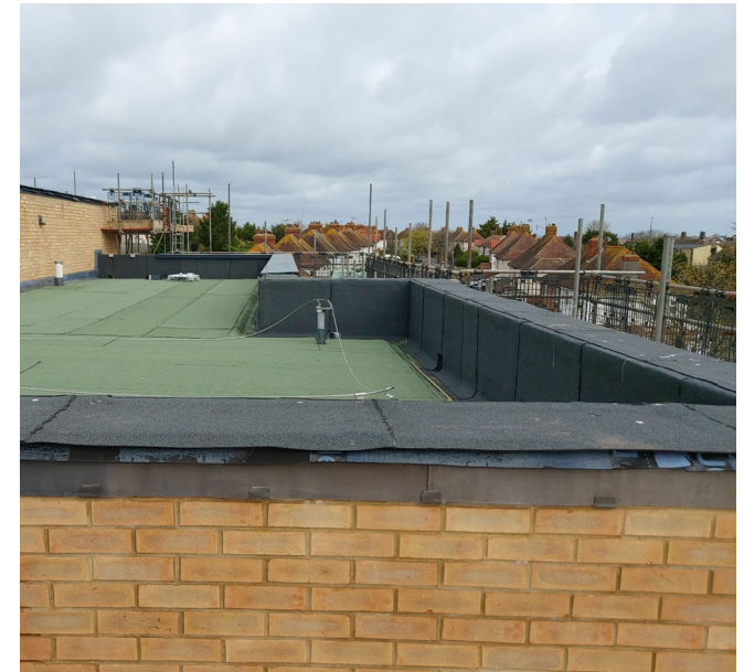
Work on going to a built-up felt roof installation. Parapets are fully encapsulated with the roof covering material with well-formed joints clearly exuding a consistent bead of bitumen. Lead work neatly formed on the outside edge, with uniform edge clipping. A proprietary capping system will complete the detailing.
