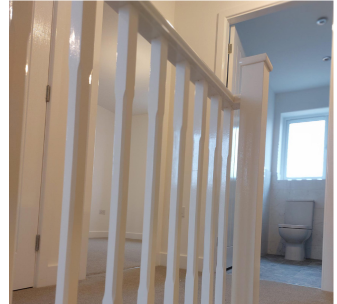
Balustrade completed with full coverage and well executed paintwork to all areas.
