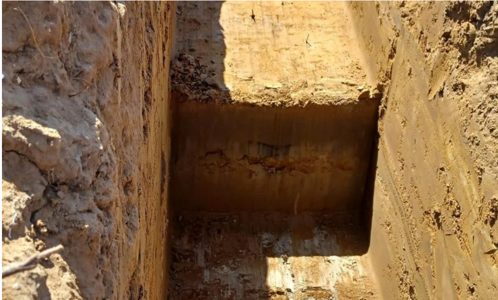
Steps in the excavation formed with accuracy and good verticality.
