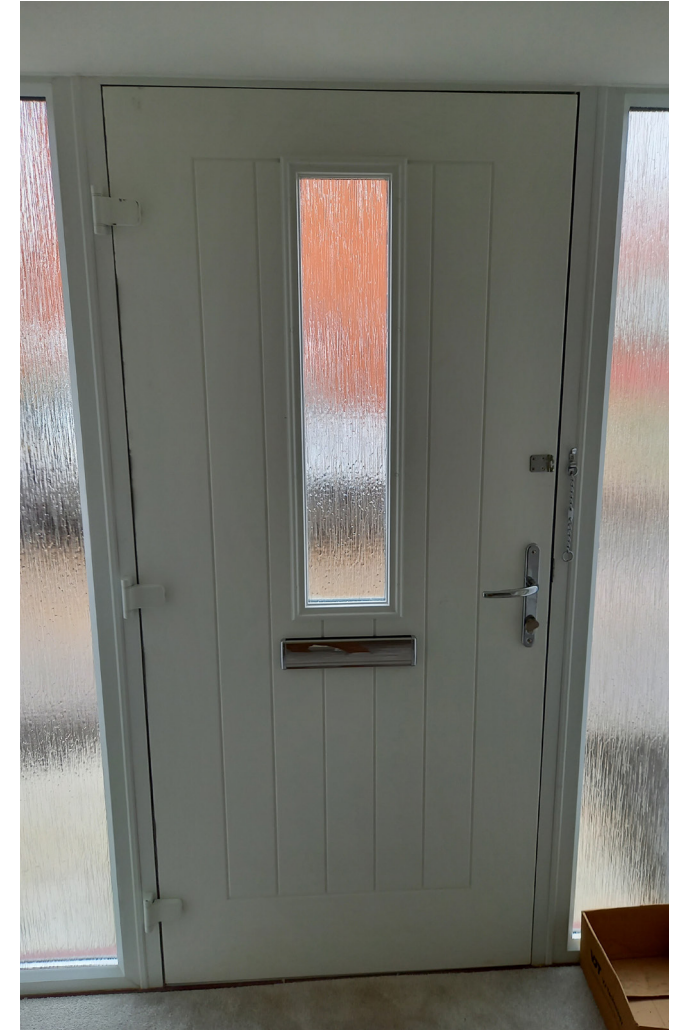
An entrance door with consistent gaps around the door leaf perimeter to ensure acceptable sealing and aesthetics.
