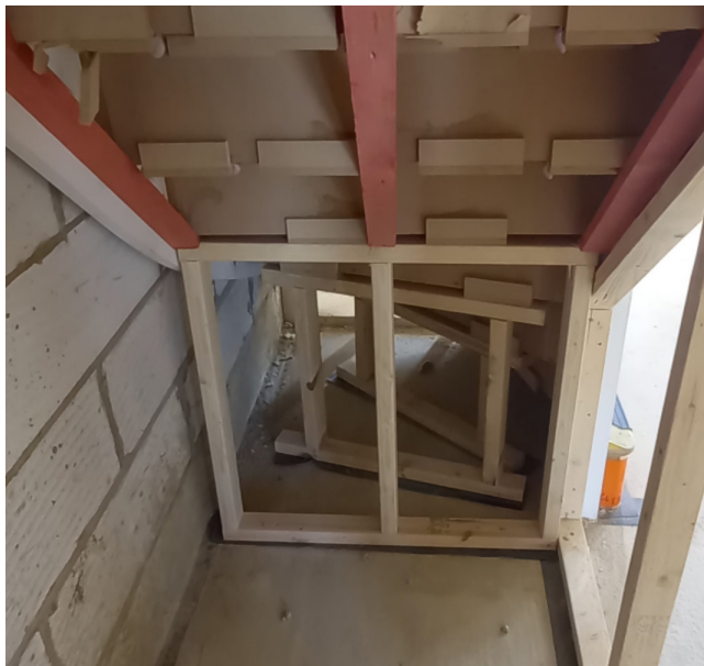
Additional timber frame installed under the staircase to support to kite winders at the base of the stair flight.
