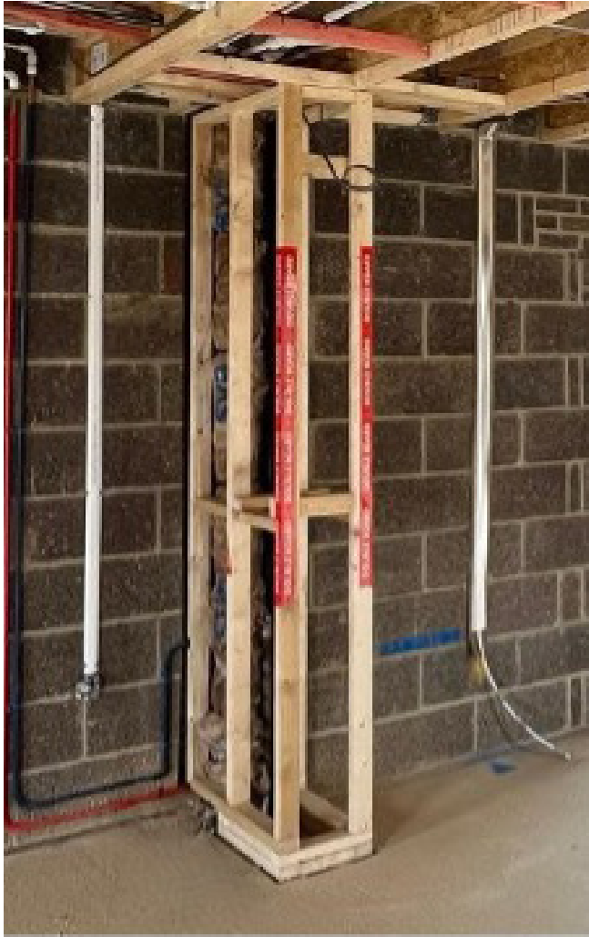
Boxing out to an SVP has been well constructed with the acoustic insulation to reduce noise transfer in place prior to construction. DPC has been placed at contact points with the wall and floor to safeguard against any residual moisture in the substrates.
