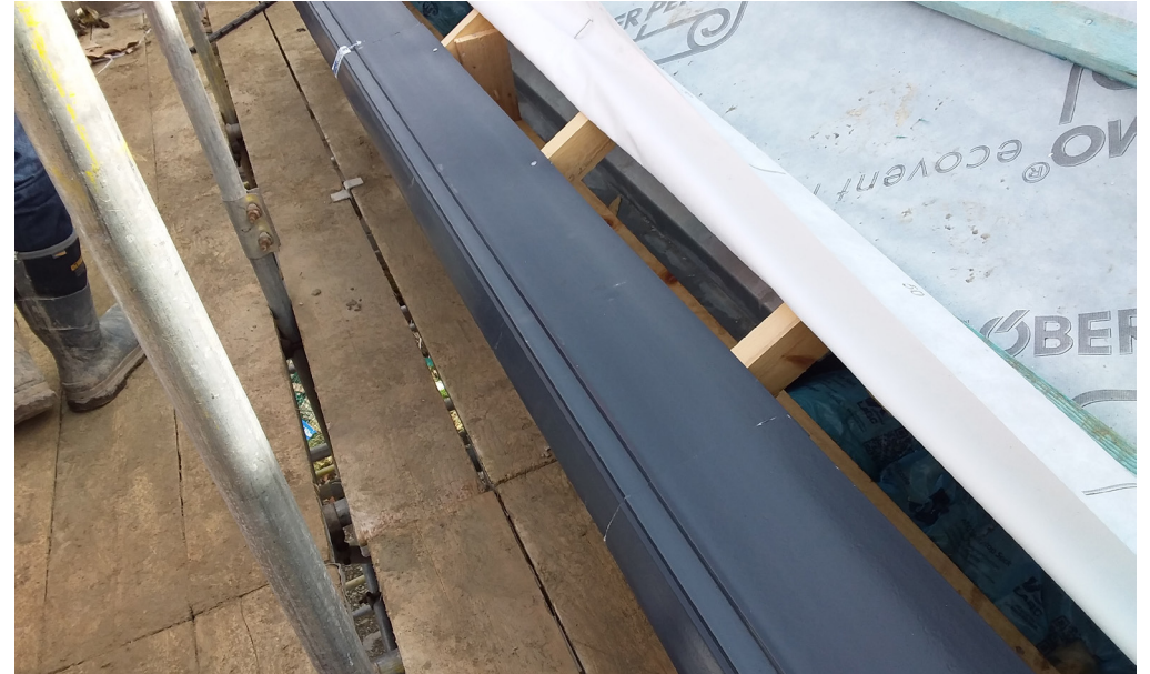
A proprietary eaves support tray installed to give full support to the underlay and ensure any water on the surface of the underlay is directed to the gutters and does not pool behind fascia boards.
