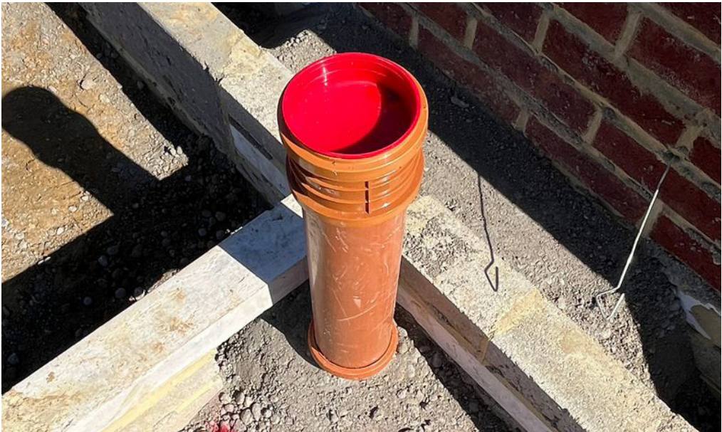
A temporary stopper inserted at a drain position to prevent construction debris accidentally entering the drain line.
