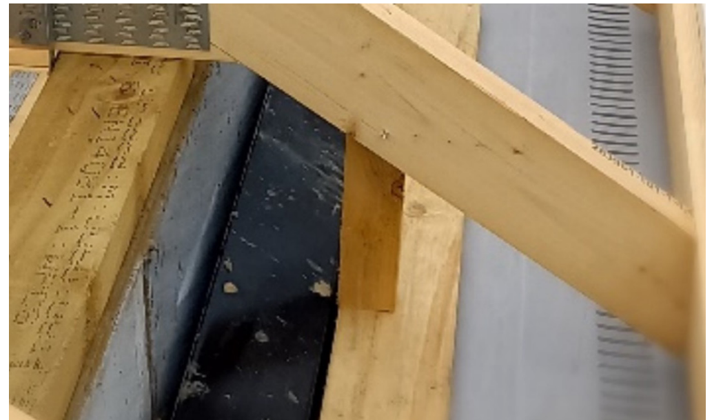
An example of well executed eaves detailing. Appropriately sized timber sections have been secured to the projecting trussed rafter end facilitating the construction of the eaves' components of fascia and ventilated soffit.
