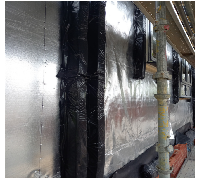
A good example of cavity fire barrier installation at a compartment wall location. Cavity fire barriers are mechanically fixed and joints are tight where they meet.
