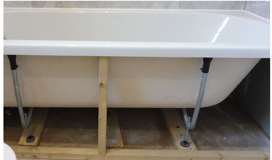
A bath installation with adjustable feet fully supported on timbers to spread the load in operation to joist positions.
