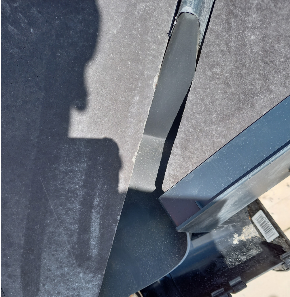
A proprietary closure unit for a GRP valley lining ensuring the valley unit is fully sealed at its end and correctly discharges into the gutter line.
