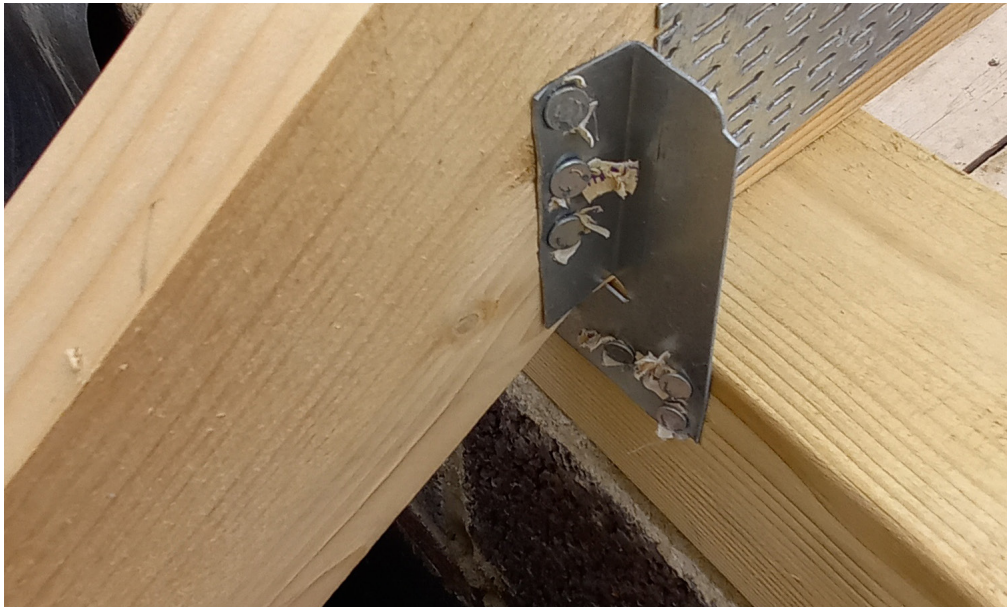
A correctly positioned trussed rafter, fully nailed and fixed using a proprietary metal bracket.
