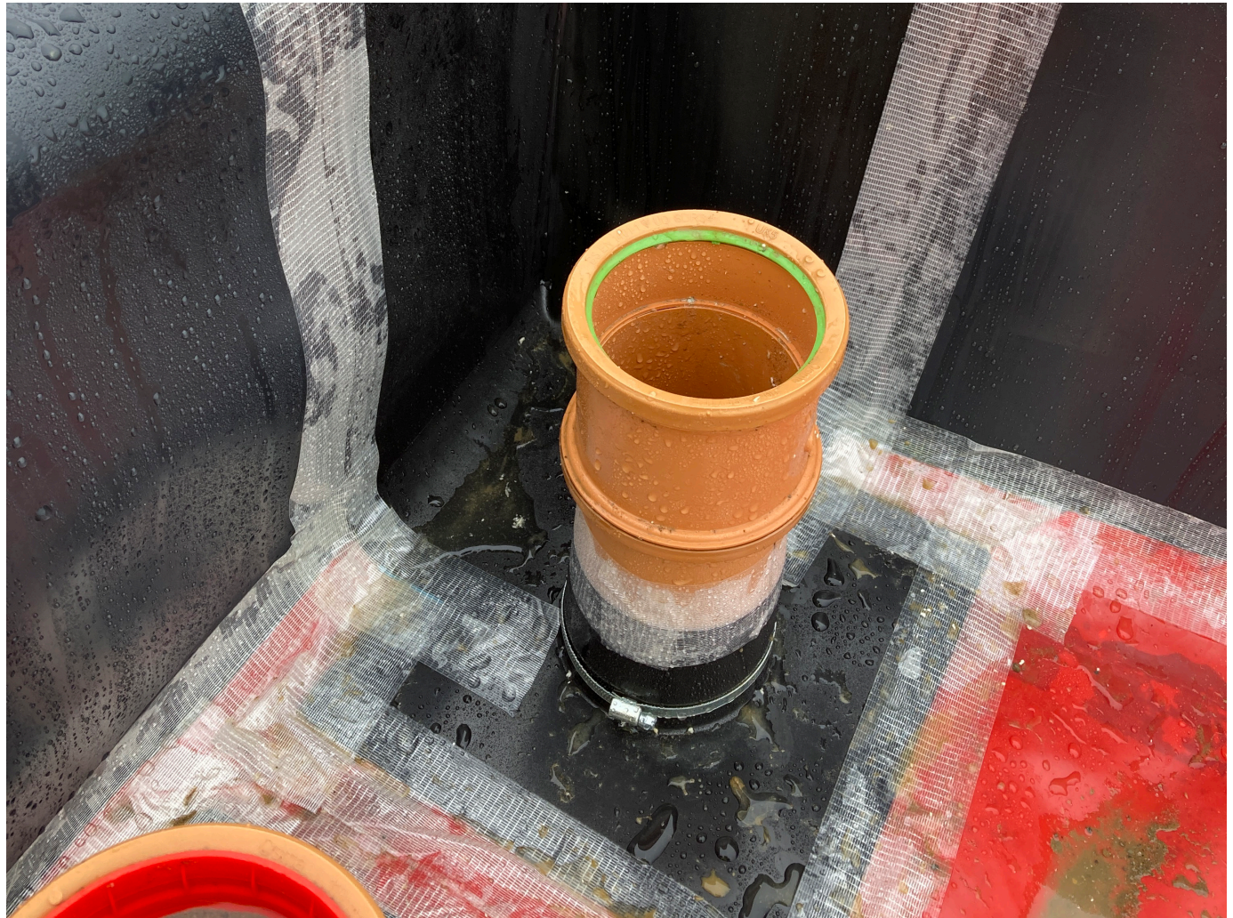
Membrane detailing with DPC has been completed to a high standard. Joints have been sealed with double sided tape and their leading edges secured with single sided tape. The membrane has been sealed to the pipe penetration using a preformed cloak, mechanically secured and its leading edge sealed.
