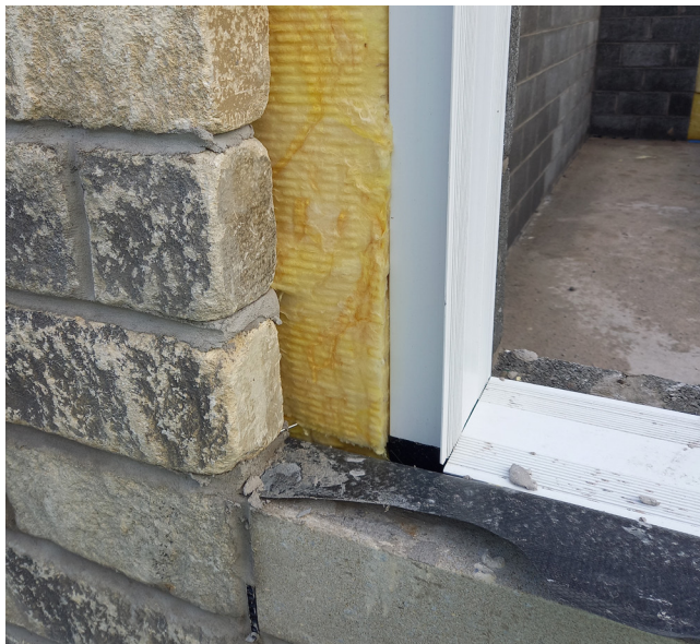
Good attention to detail around this opening with cavity insulation being finished tight into the closure unit prior to the follow-on stone surround work commencing.
