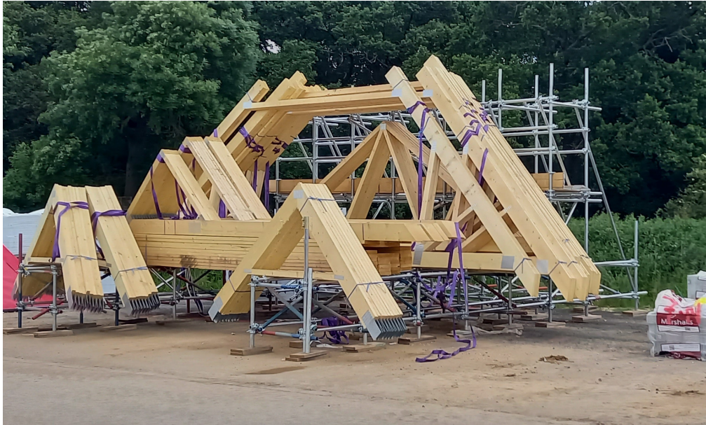
An example of a well-arranged trussed rafter storage area. Stored securely and off the floor, the trussed rafters avoid damage and soiling from surrounding site operations.
