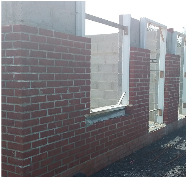
Proprietary thermal cavity closure units being built into openings. Bracings have been applied at corners and across the openings to ensure they maintain an accurate shape.
