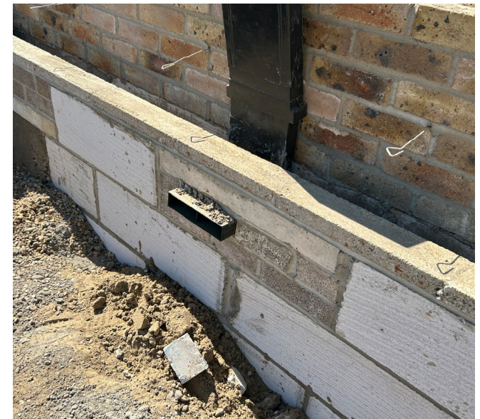
Splash courses being brought up to level – good clean jointing to the cavity face. The telescopic vent is positioned to course in with external masonry and the penetration is now neatly closed with no gaps or voids.
