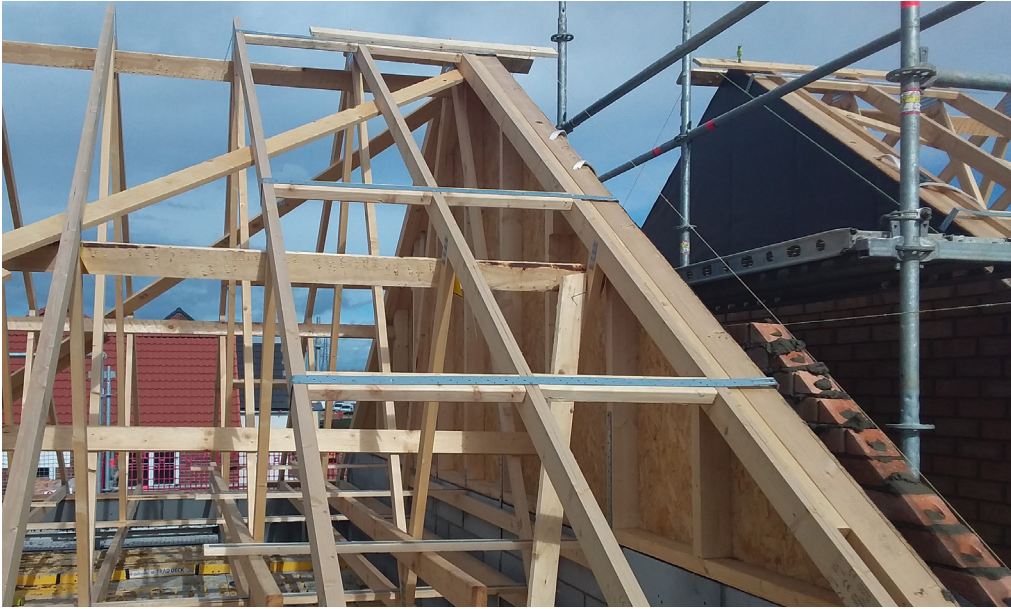
Lateral restraint is provided by means metal restraint straps. These are within the 2m maximum centres and correctly fixed over 3 trussed rafters and bracing timbers and turned down the face of the spandrel panel.
