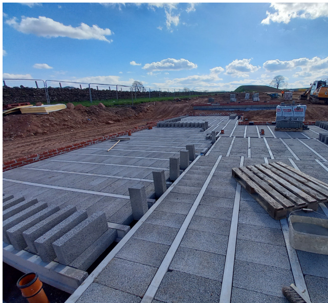
Block infill work in progress - all beams are placed tightly against the blocks. Neatly cut units are being readied for placement.
