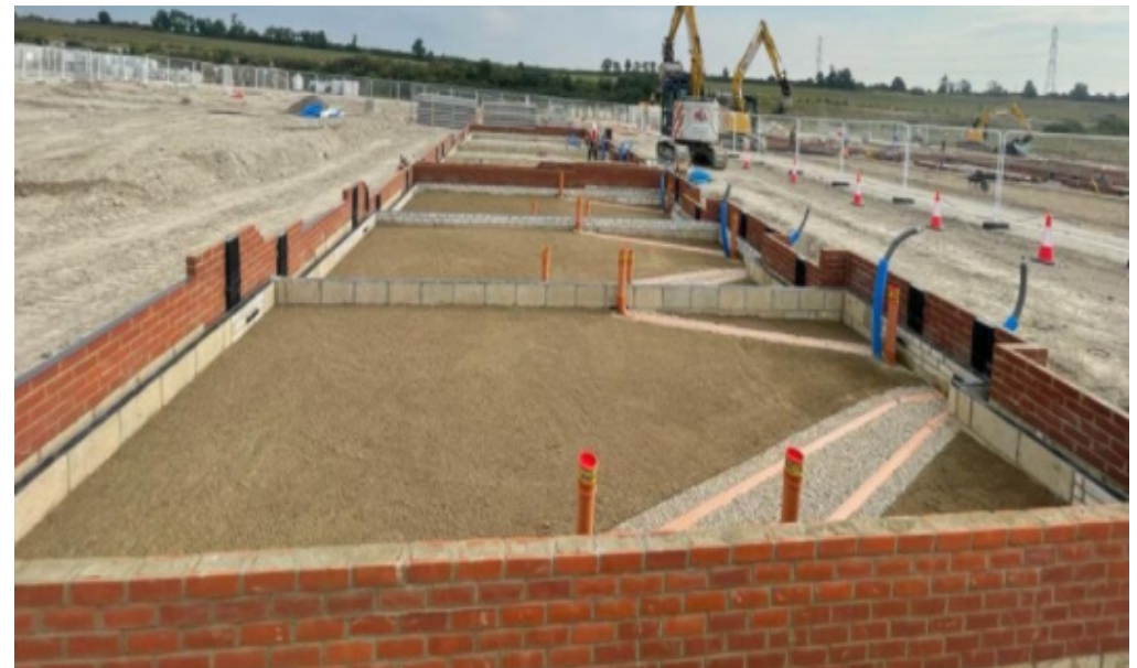
Well set out sub-floor drainage runs, supported on well graded pipe bedding material with good lines and sufficient falls. Work area cleared and ready for inspection.
