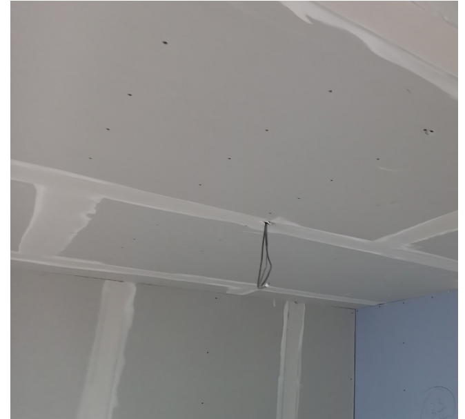
Uniform and correctly spaced screws securing the ceiling plaster boarding.
