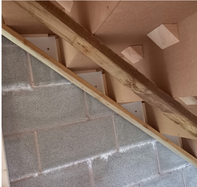
The wall string firmly secured to the adjacent wall using frequently spaced fixings.
