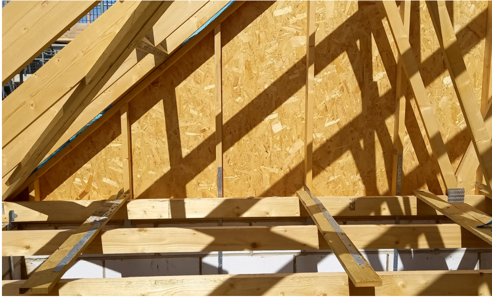
This gable spandrel panel has horizontal proprietary metal twist straps fixed onto longitudinal bracing and into vertical studs within the panel alongside vertical strapping down to the masonry below.
