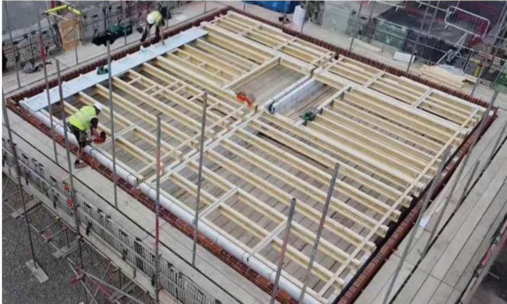
A completed intermediate engineered timber joist floor and the commencement of structural floorboard installation.
