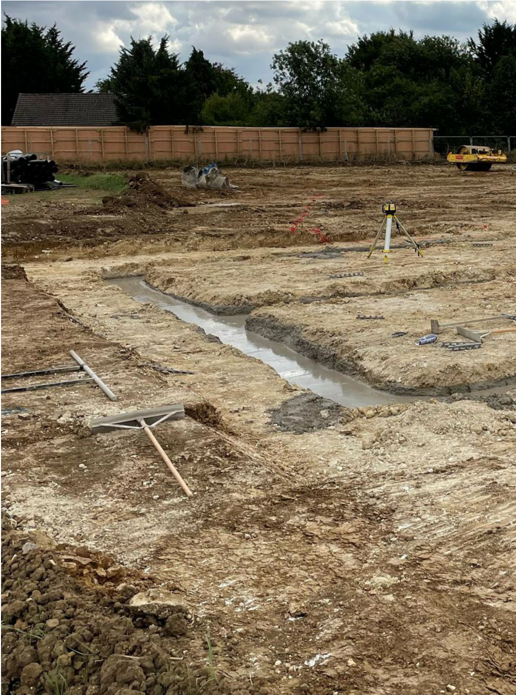
Controlled finishing being executed to achieve a good level surface for follow-on substructure masonry.
