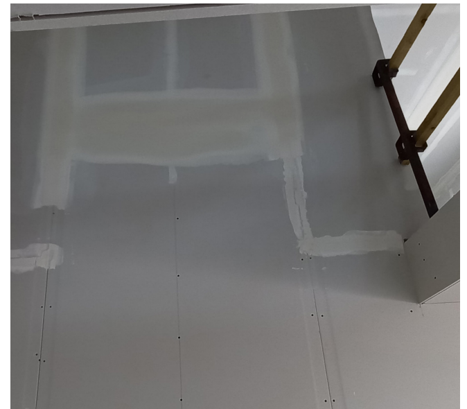
Tape and filling work ongoing to these staggered joints formed in this two-storey high wall. Staggering horizontal plaster board joints reduces the risk of horizontal linear cracking.
