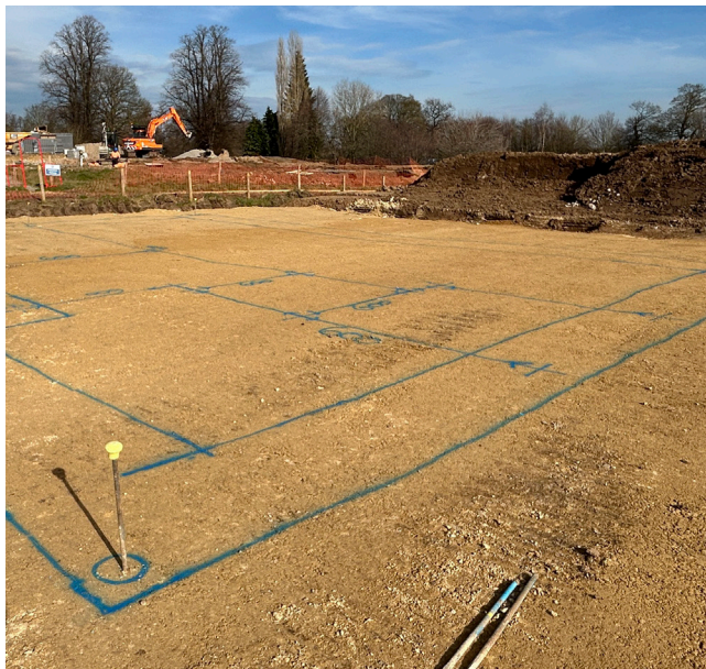
A plot marked out in readiness for excavation activity. Levelled, accessible and clear.
