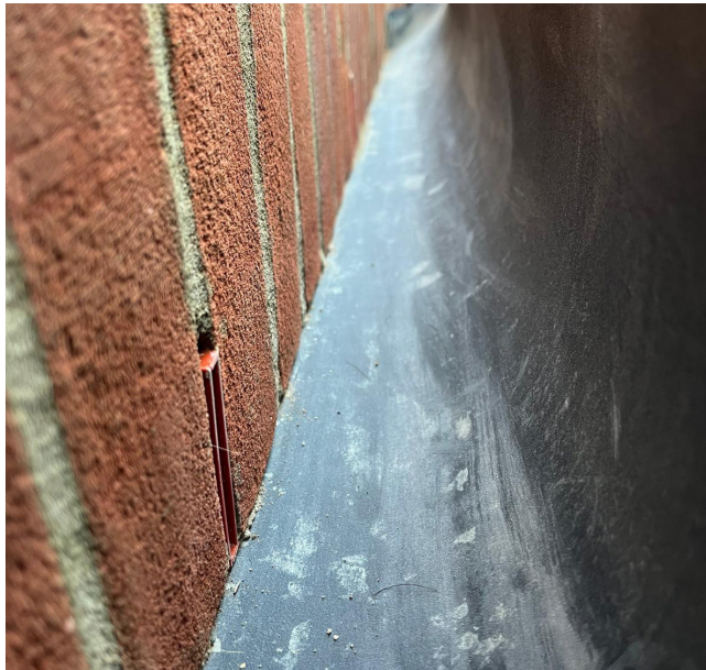
External masonry leaf to timber frame with a clean cavity tray. Ventilation and drainage of the cavity facilitated by a series of weep vents within the vertical perpendicular mortar joints in the soldier course.
