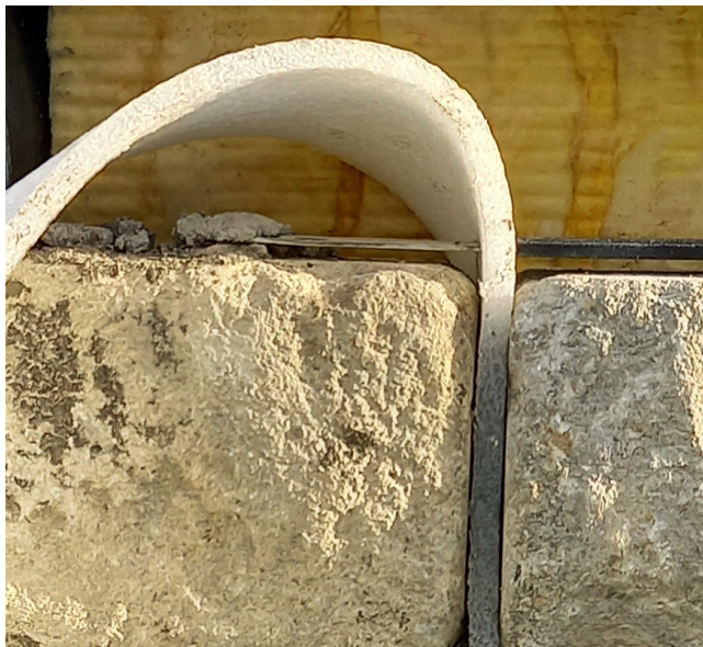
Proprietary slip ties built into the masonry panel movement joint. Compressible polyurethane foam has been neatly placed, and a debonding sleeve in place ready to be embedded in mortar.
