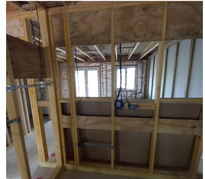
Uniformly executed pattress work to facilitate the fixing of kitchen cabinets. Again, timber grounds have been correctly included to facilitate squarely driven fixings to ensure the element of support is well secured.
