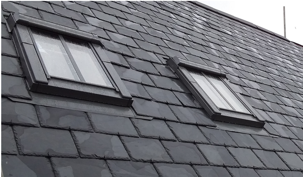
A well-presented rooflight installation. Proprietary flashing kits have been used and the bottom apron flashing aligns well with adjacent slate coursing. Cut work is neat and tidy and the slate termination detailing into the rear of the flashing kits observes the required gap.
