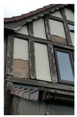
This image to the left demonstrates what can go wrong, in this instance the timber has been planted onto the external masonry cavity wall and the panels rendered in between. Movement in the timber then leads to water ingress behind the render and premature failure of the render system.
