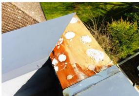
Image top left represents a situation where the DPC and DPC support has been omitted. As a result mortar bedding is not present and the copping has detached. Image top right represents a situation where the DPC has been omitted and the capping has been attached using mastic. Adhesion has failed and the lack of mechanical fixing has resulted in detachment and water ingress.
