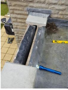
Failures in the horizontal DPC are common place. In the image to the left, we can identify a DPC of incorrect width, a lack of support to the DPC as it crosses the cavity and a lack of sealed joints in the DPC. The image to right shows a complete omission of the DPC, which has compounded the cavity tray issue (described below).
