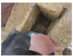
Images depict a raking parapet with stone copings. Various failings of the 3 lines of defence are present such as a horizontal DPC of incorrect width which lacks support across the cavity, a lack of mortar bedding across the full width of the wall and missing mechanical fixings leading detachment of the coping, and the omission of the cavity tray.
