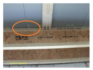
• Lack of edge gap between floor deck and solid walls:
