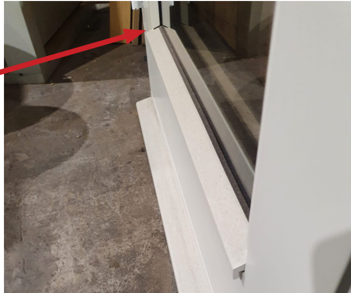
Image showing correctly scribed beading
