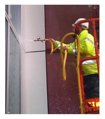
Most systems that have passed a laboratory static water-tightness test at 600 Pa, including many with opening joints, should pass an on-site hose test at full water pressure so long as the details, materials and workmanship are the same as tested in the laboratory.
