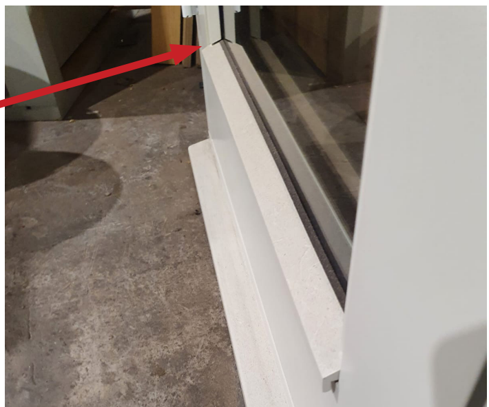
Image showing correctly scribed beading
